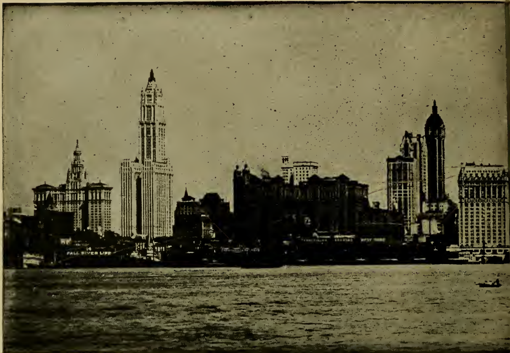
Municipal. Woolworth. Am. Tract Soc. Western Union. City Investing. Columbia. Tribune. Park Row. Hudson Terminal. Singer.
