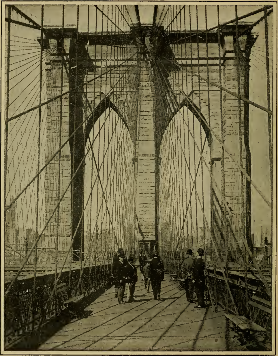
THE MANHATTAN TOWER OF THE BROOKLYN BRIDGE.
