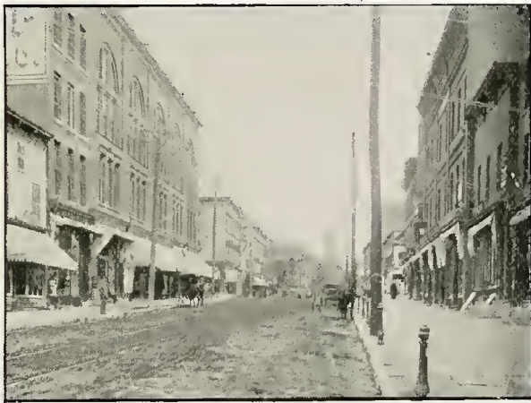
CHURCH STREET, Looking North.
