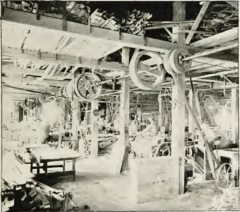
VENETIAN BLIND COMPANY'S SHOP.
