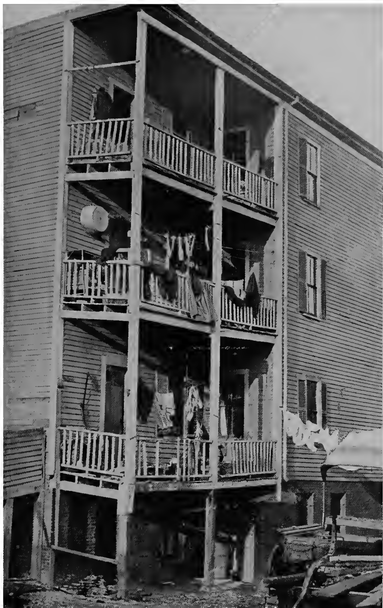
Rear view of a typical three-decker.
