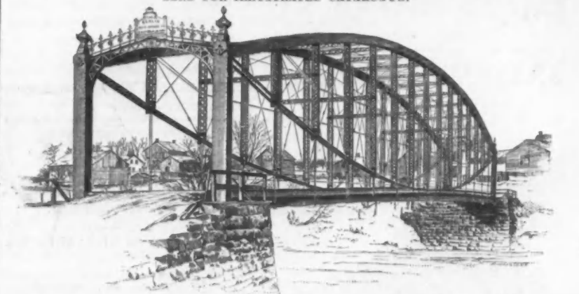
THE above illustration, taken direct from a photograph, shows the construction of an Iron Truss Bridge, designed and built by us at Massena, St. Lawrence County, N. Y., consisting of one span of 235 feet with a roadway 16 feet wide in the clear.
