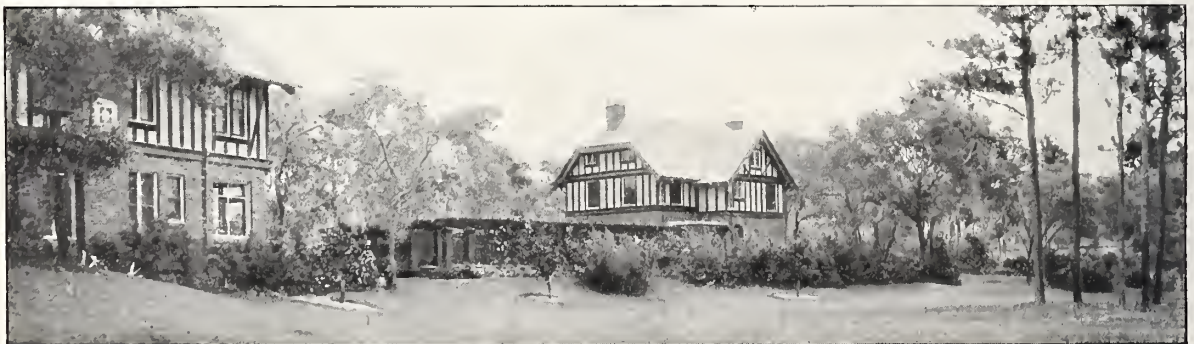
Screening the garage and lending an atmosphere of distance
