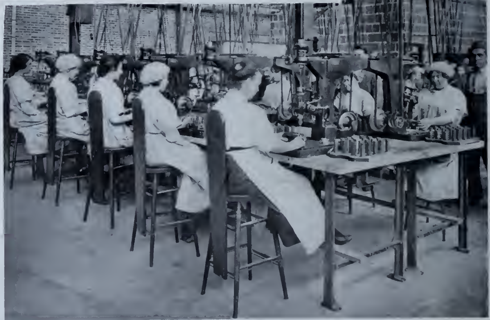
Drilling Holes Preparatory to Routing the Powder Groove, No. 80 Fuse
