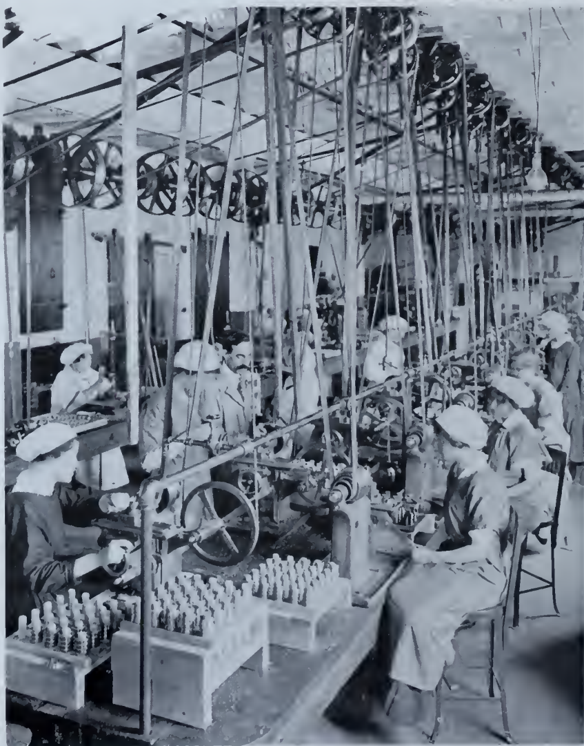
Various Milling Operations on Top and Bottom Rings No. 80 Fuse
