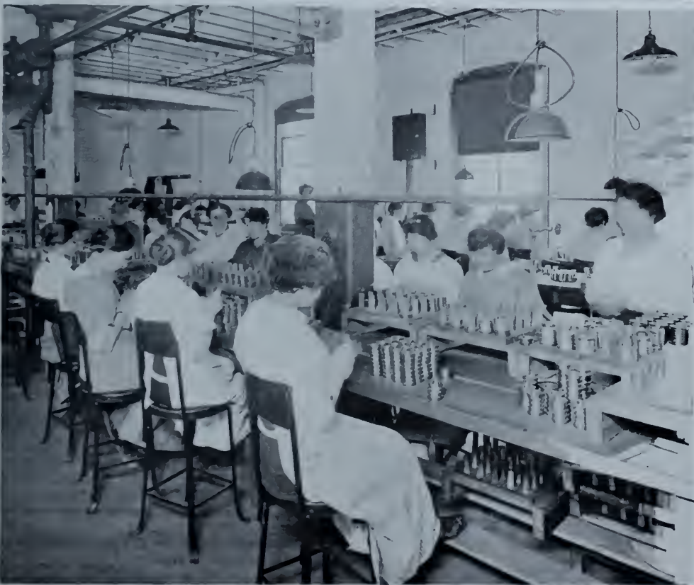
Inspection of Top and Bottom Rings No. 80 Fuse
