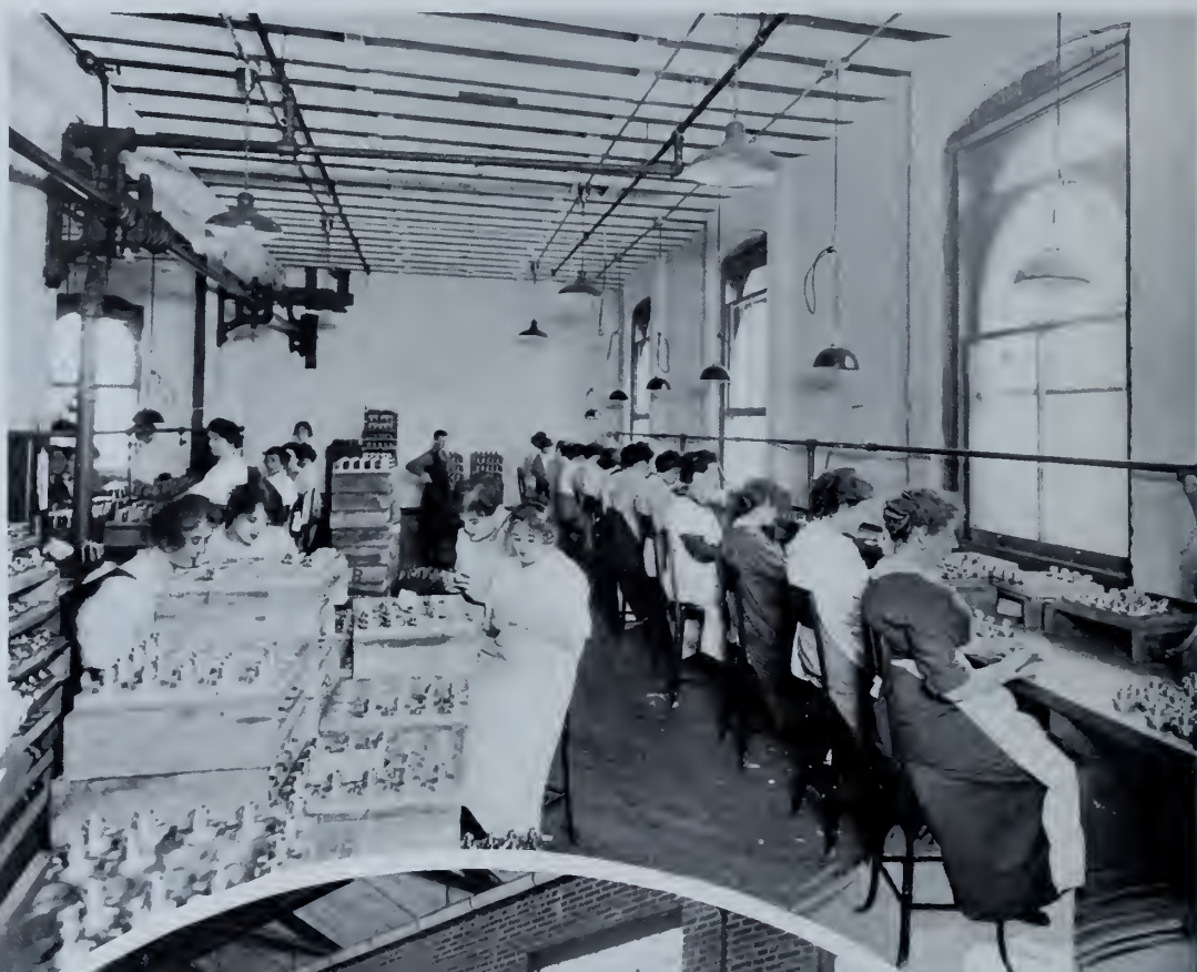
Inspection of Bodies No. 100 Fuse
