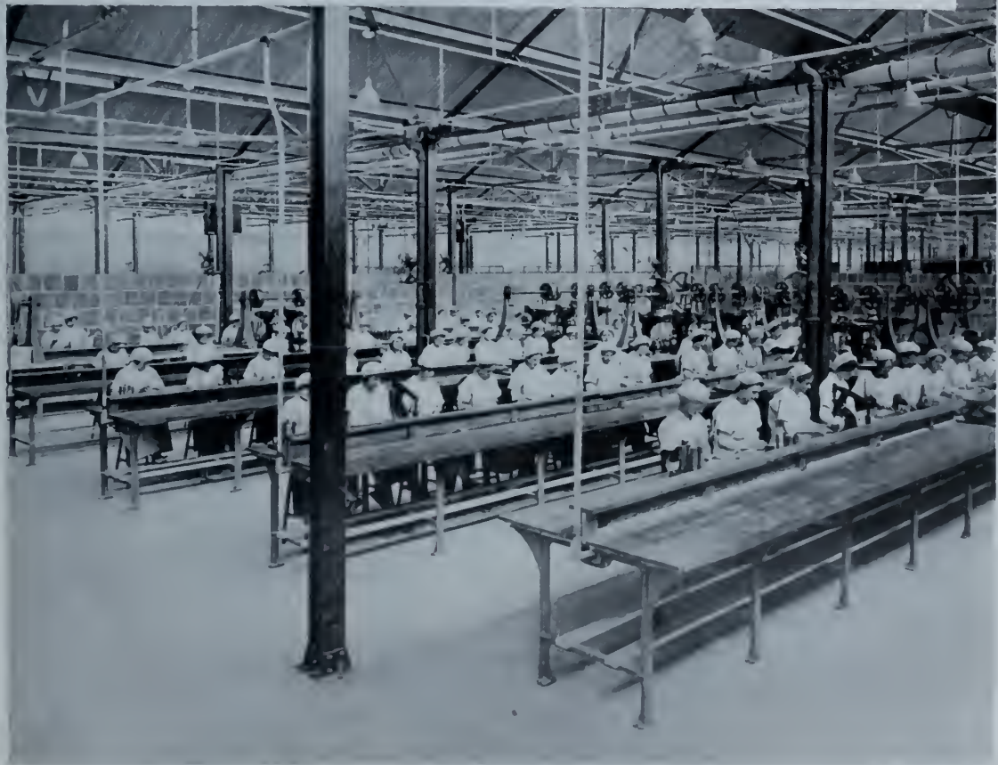
General Views of Assembly Room, No. 80 Fuse
