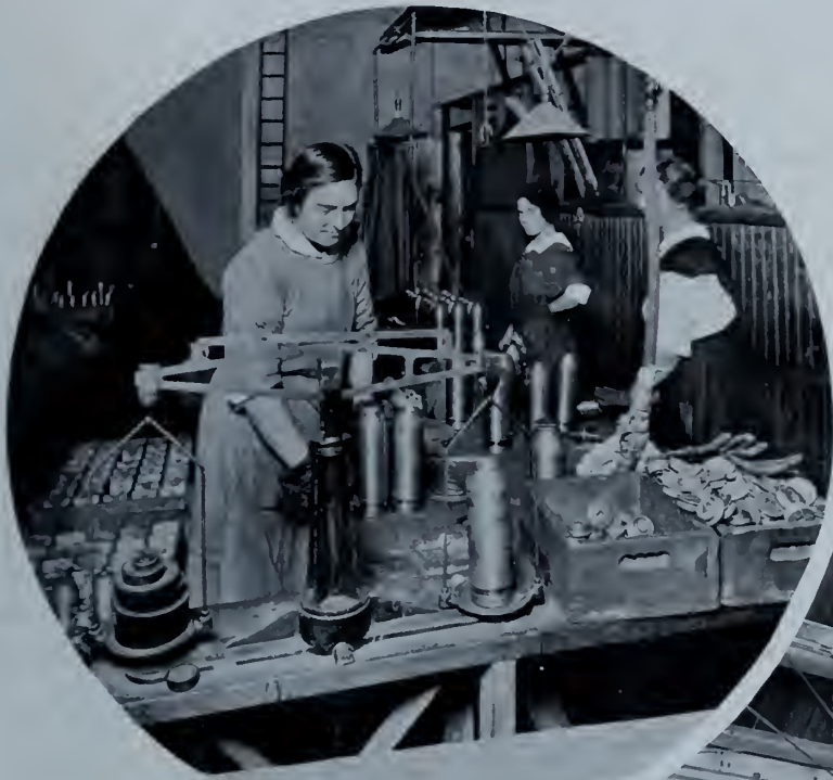
Swabbing Out Tubes and Weighing
