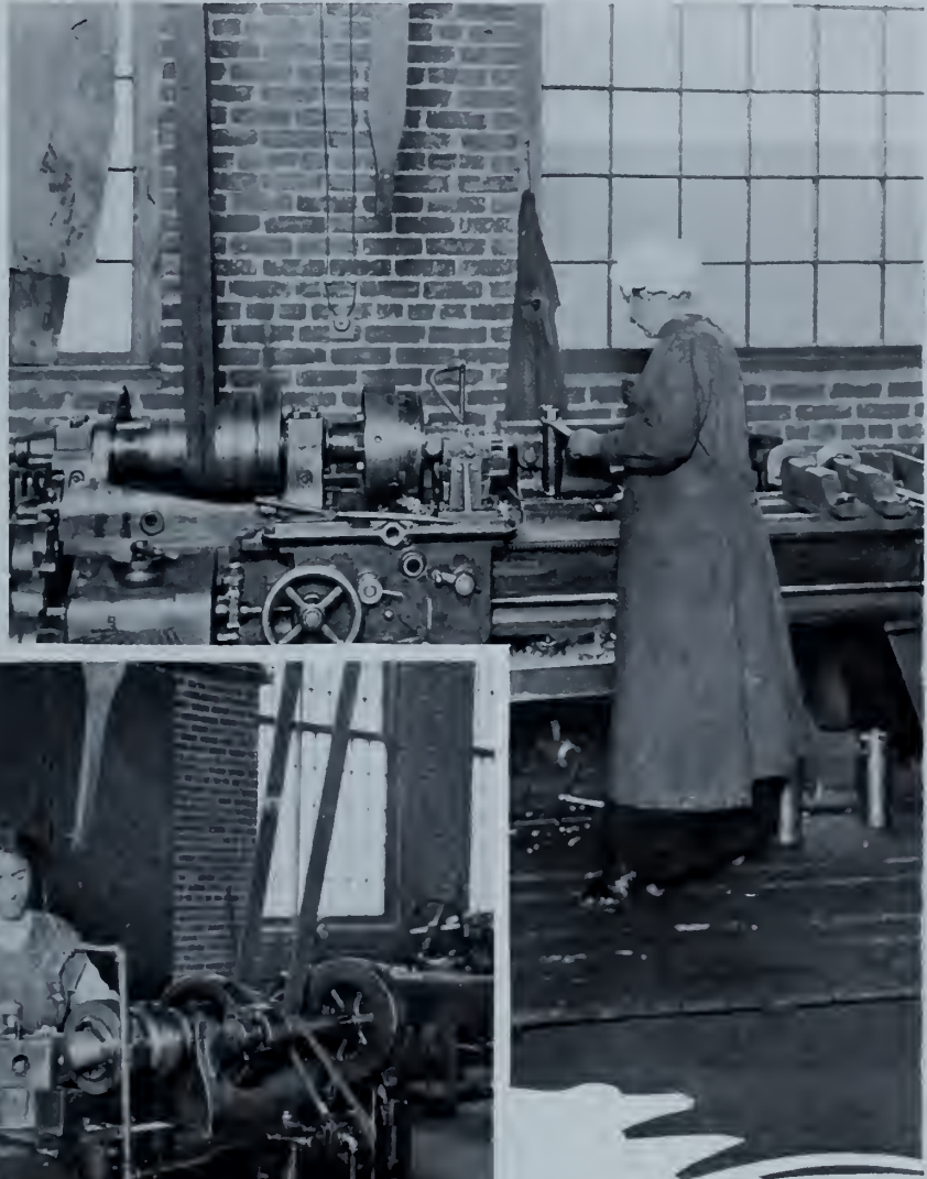
Waving and Undercutting for Copper Band, 18-pounder Shrapnel
