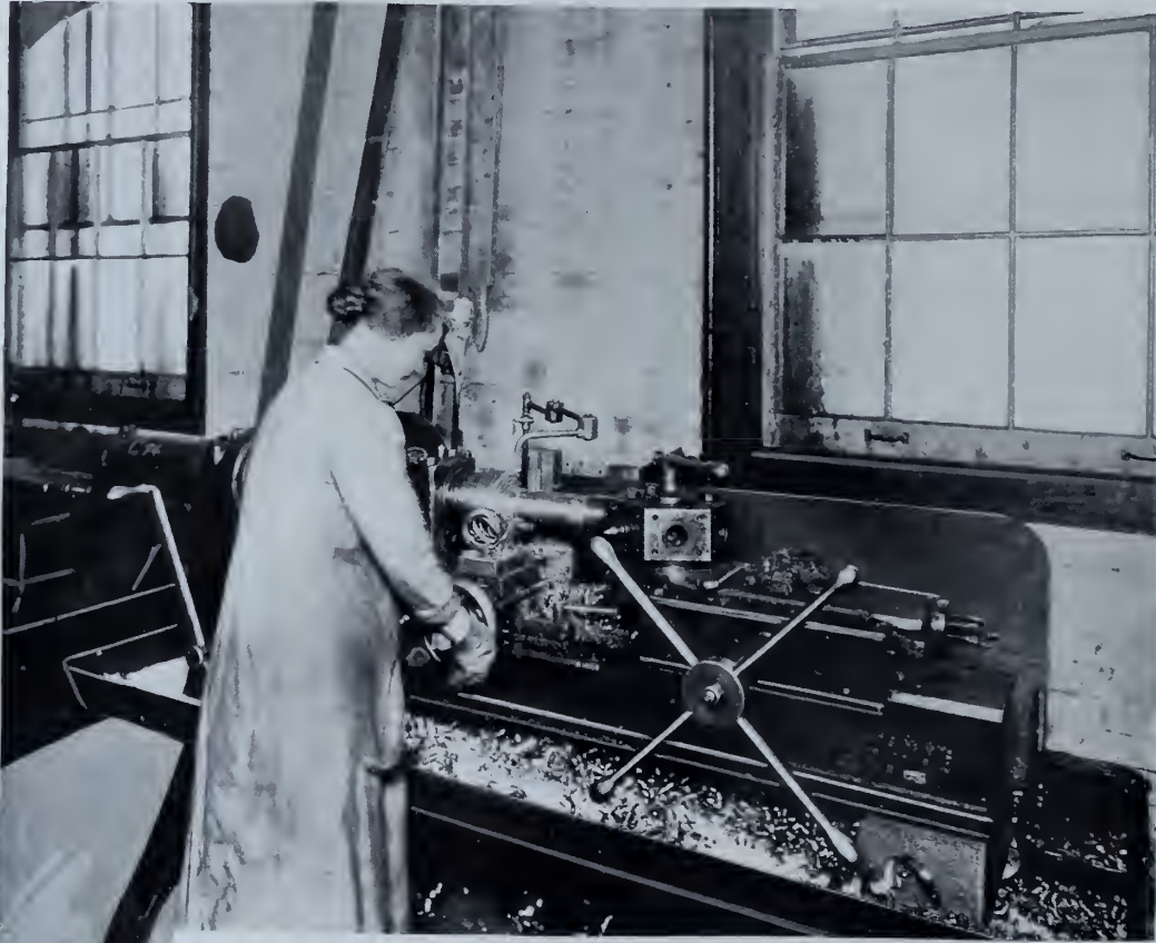
Turning Copper Driving Band
