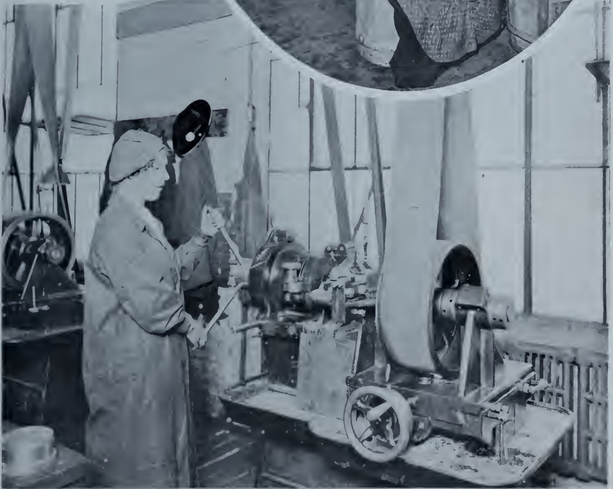
Milling Thread on Adaptor for 8 inch Shells
