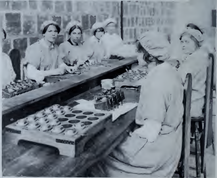
Close Operation of Filling the Base Charge No. 80 Fuse
