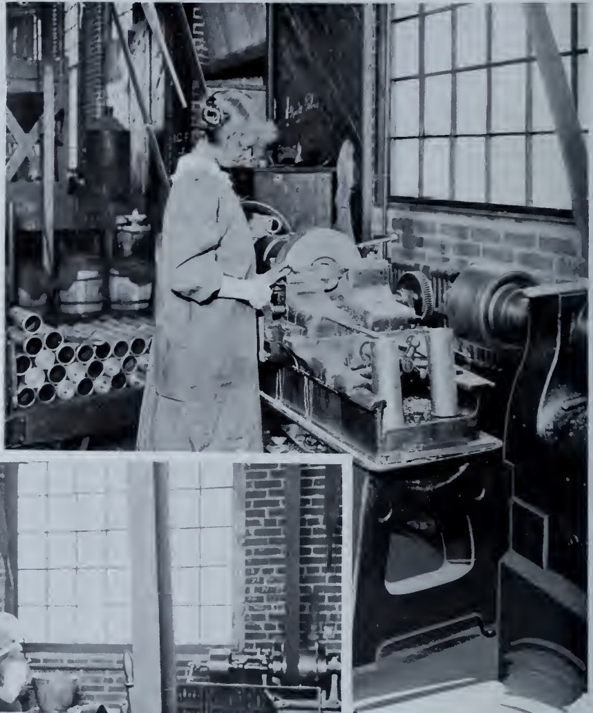
Cutting Off the Base 18-pounder Shrapnel
