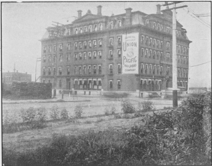
22.—The Union Pacific Building, Omaha,—site of one of the “jumping off” points for Oregon.
