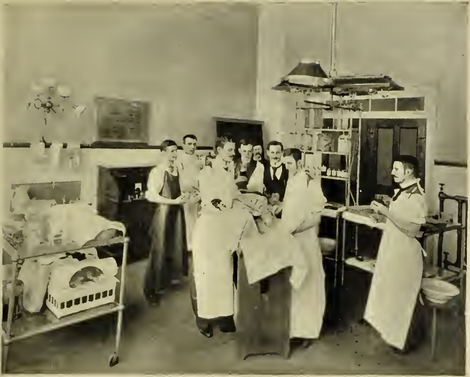
Crane Operating Room.
