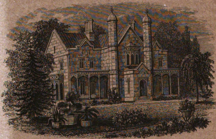
RESIDENCE OF A. J. DOWNING, ESQ. NEWBURGH, N. Y.
