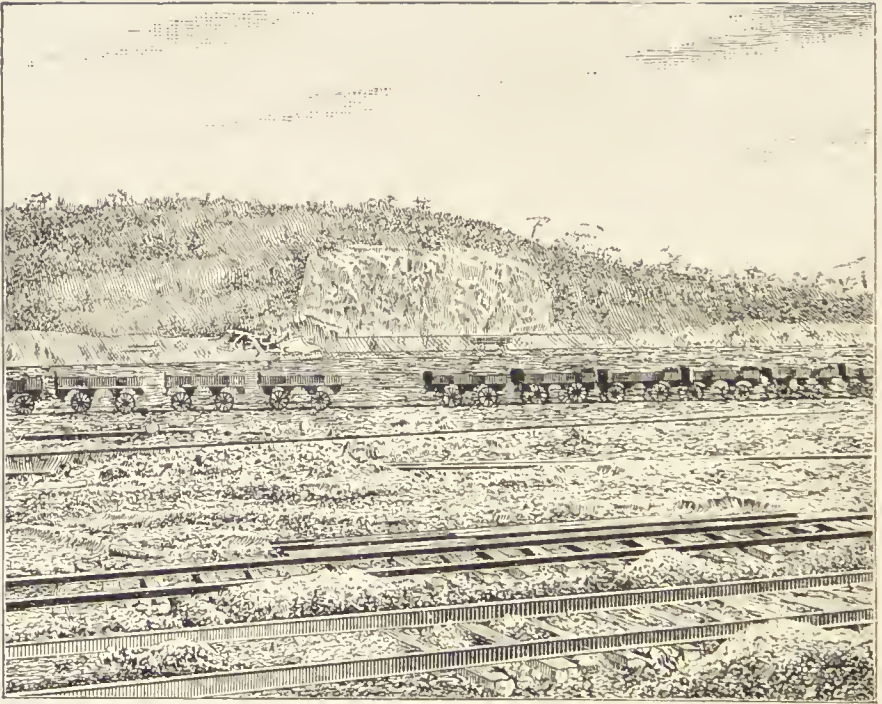
CANAL CUT AT EMPERADOR ; 187 FEET ABOVE SEA-LEVEL.
