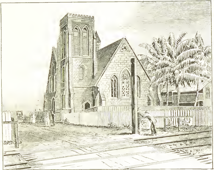
EPISCOPAL CHURCH, COLON; BUILT BY PANAMA RAILWAY.
