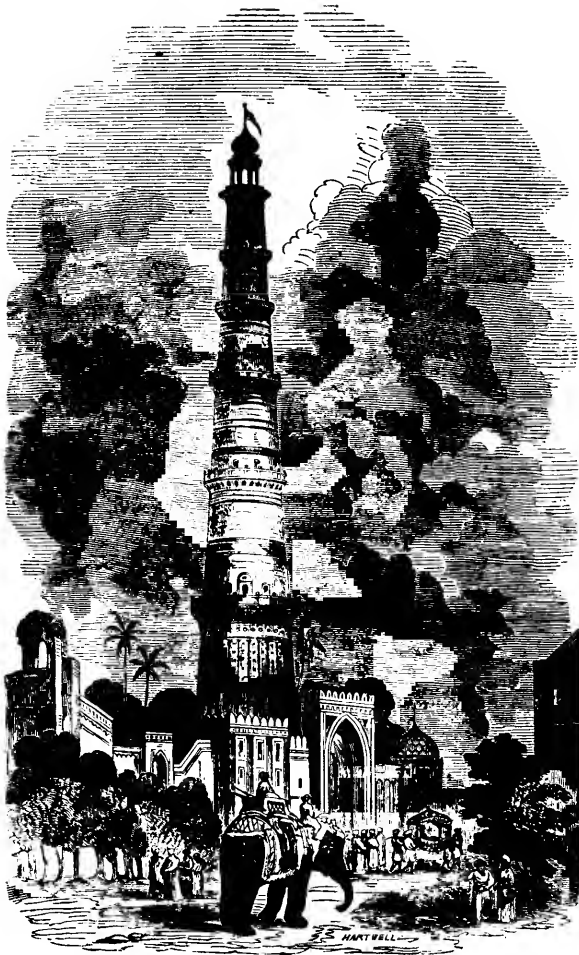
The great Minaret at Delhi. Its height is 242 feet. In the interior is a spiral staircase leading to the different balconies and to the top. It was built in the thirteenth century, but for what purpose is now unknown.
