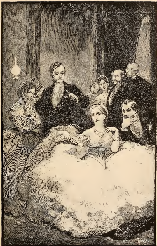
FIG. 7—HOME AT THE TUILERIES,
