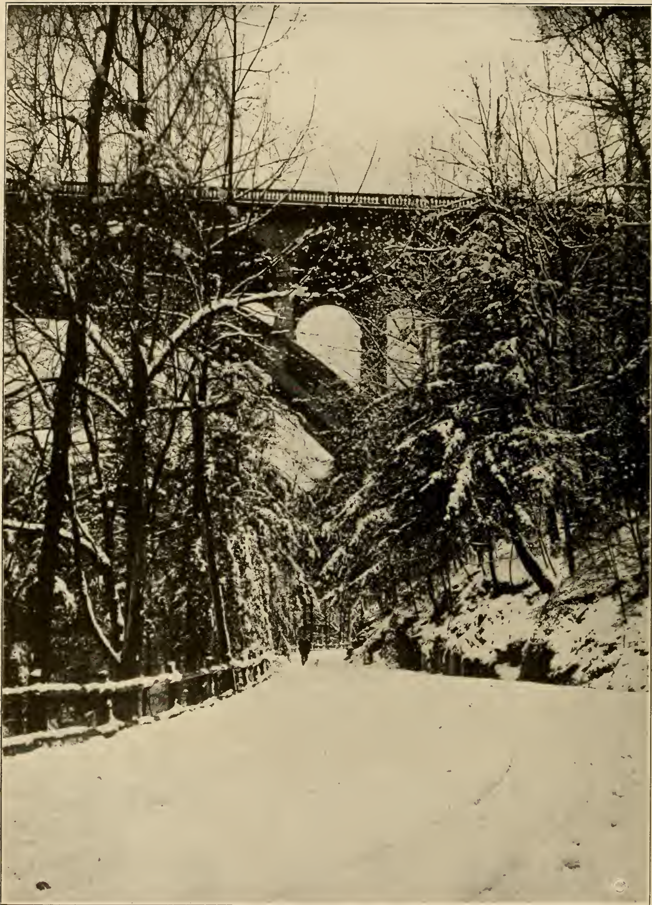
WESTERN END OF WALNUT LANE BRIDGE, WISSAHICKON DRIVE.
