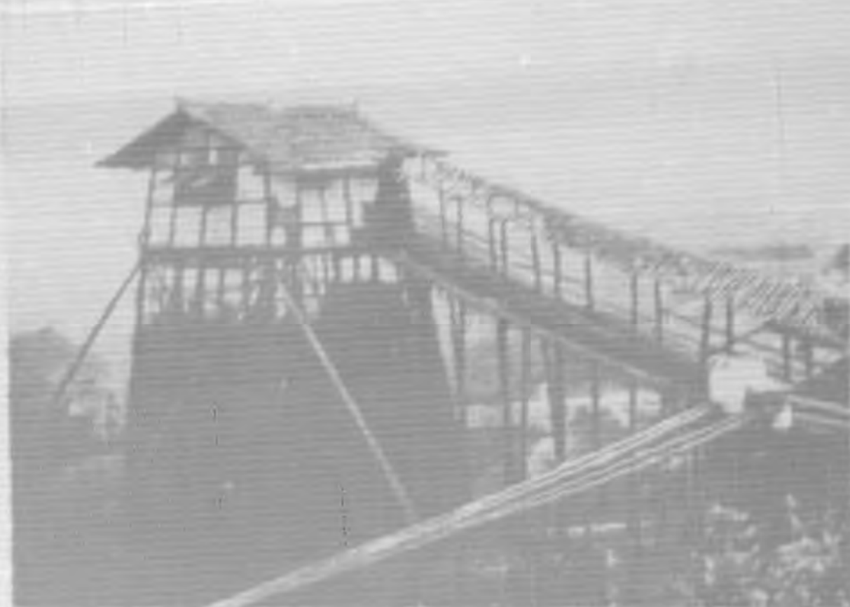
自流井貢井區視檢視高 Pipe line towers and junctions in the Tzuluchung-Kuogching region,
