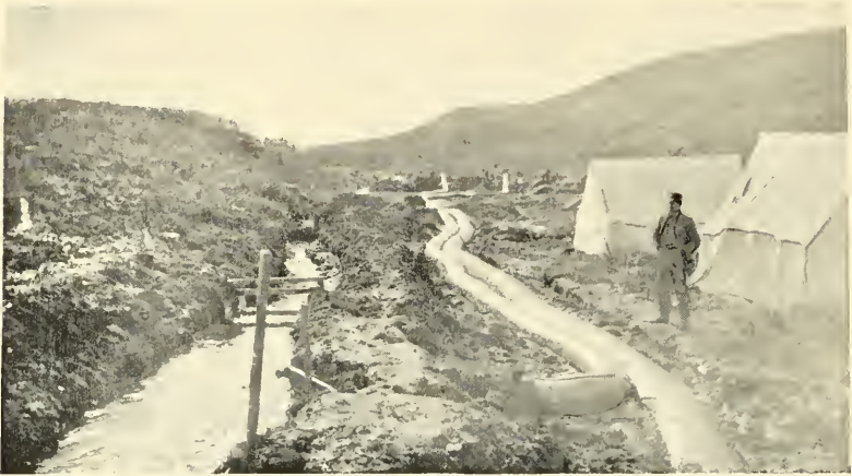
SHOWING DAM DRAIN AND A FEW LENGTHS OF CANVAS HOSE ON CLAIM NO. 5, ABOVE, ON ANVIL CREEK.
