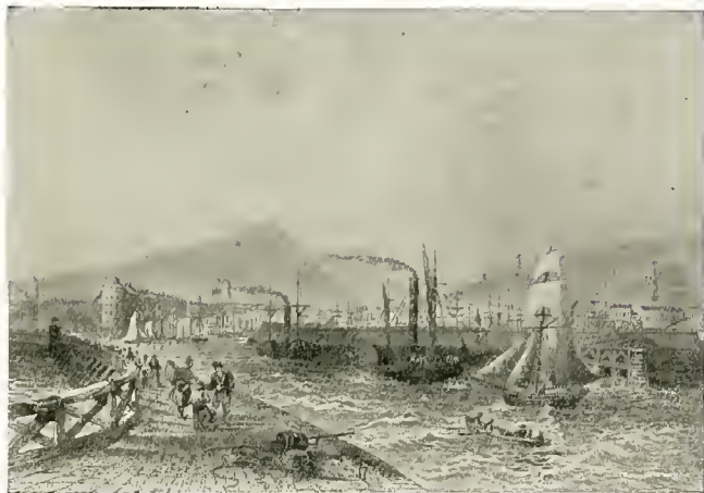
Leith Pier and Harbor.
