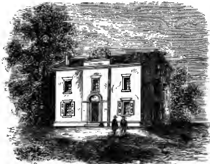
ARSENAL BUILDING, WATERTOWN.
