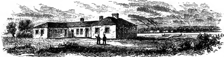
BARRACKS AT SANDWICH.
