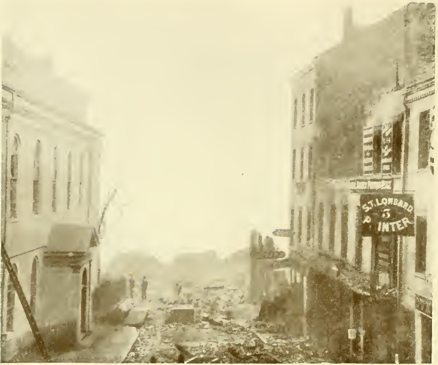
LOOKING DOWN FROM MILK STREET, FROM WASHINGTON STREET AFTER THE GREAT FIRE OF 1872
