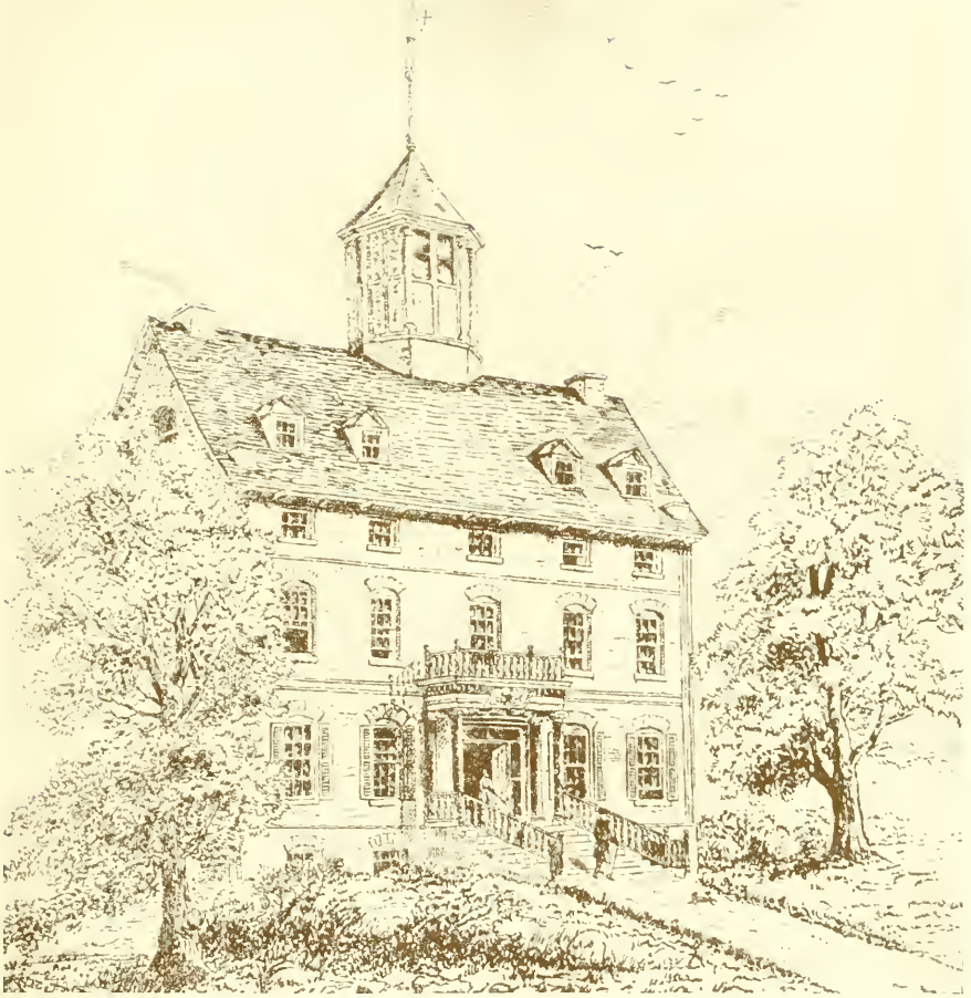
THE PROVINCE HOUSE, ON THE WEST SIDE OF WASHINGTON STREET, PRESENT SITE OF PROVINCE COURT
