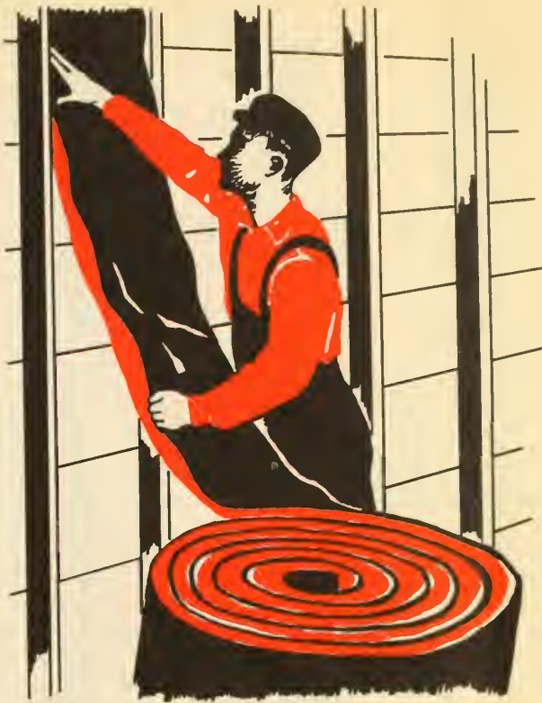
Figure 14.—Blanket insulation fits between joists.
