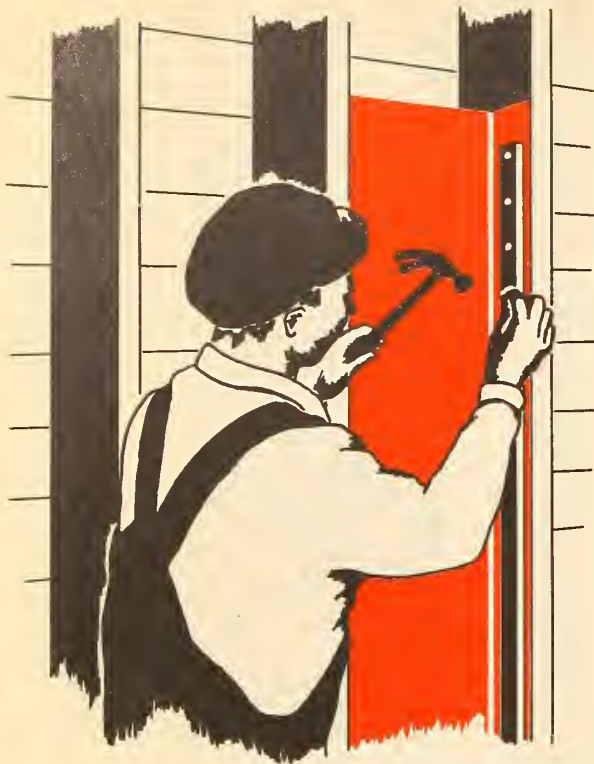
Figure 16.—Reflective insulation adds to comfort in southern homes.
