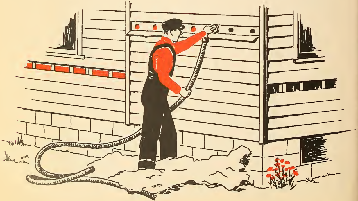
Figure 13.—Loose-fill insulation is poured into place.
