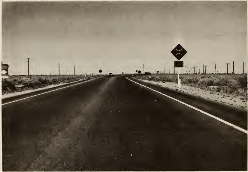
Figure 49 Primary Sign and Message Plate (Santa Fe Crossing)
