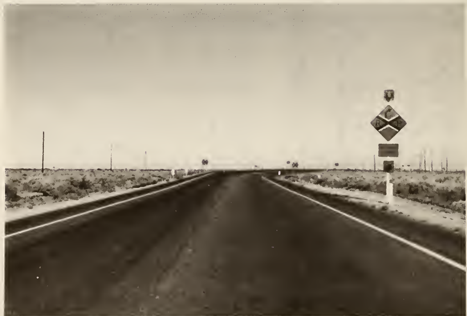
Figure 50 Activated Advance Warning Device (Santa Fe Crossing)
