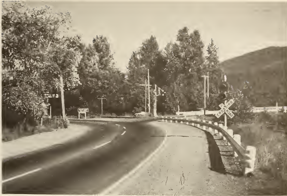
Figure 5 Washington State Installation
