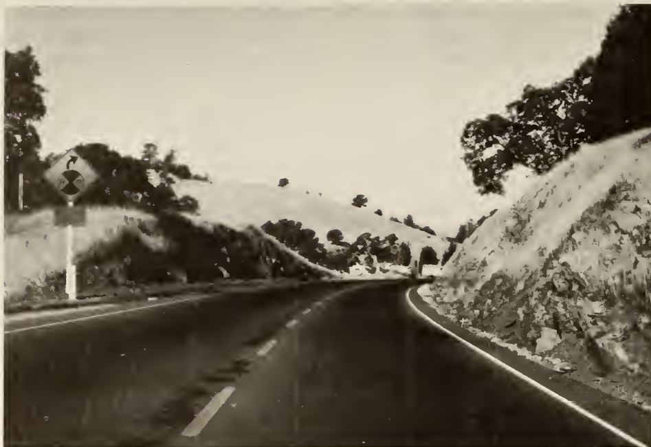
Figure 59 Primary Sign C And Supplemental Message (Amador Central Crossing)
