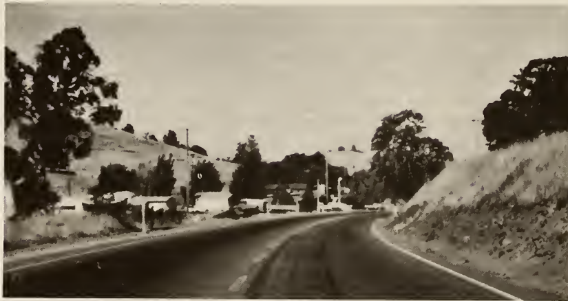
Figure 53 Driver View - 1200 Feet (366m) (Amador Central Crossing)
