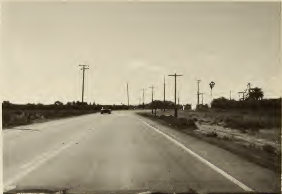
Figure 66 Pole Clutter (With dark background framed signals)
