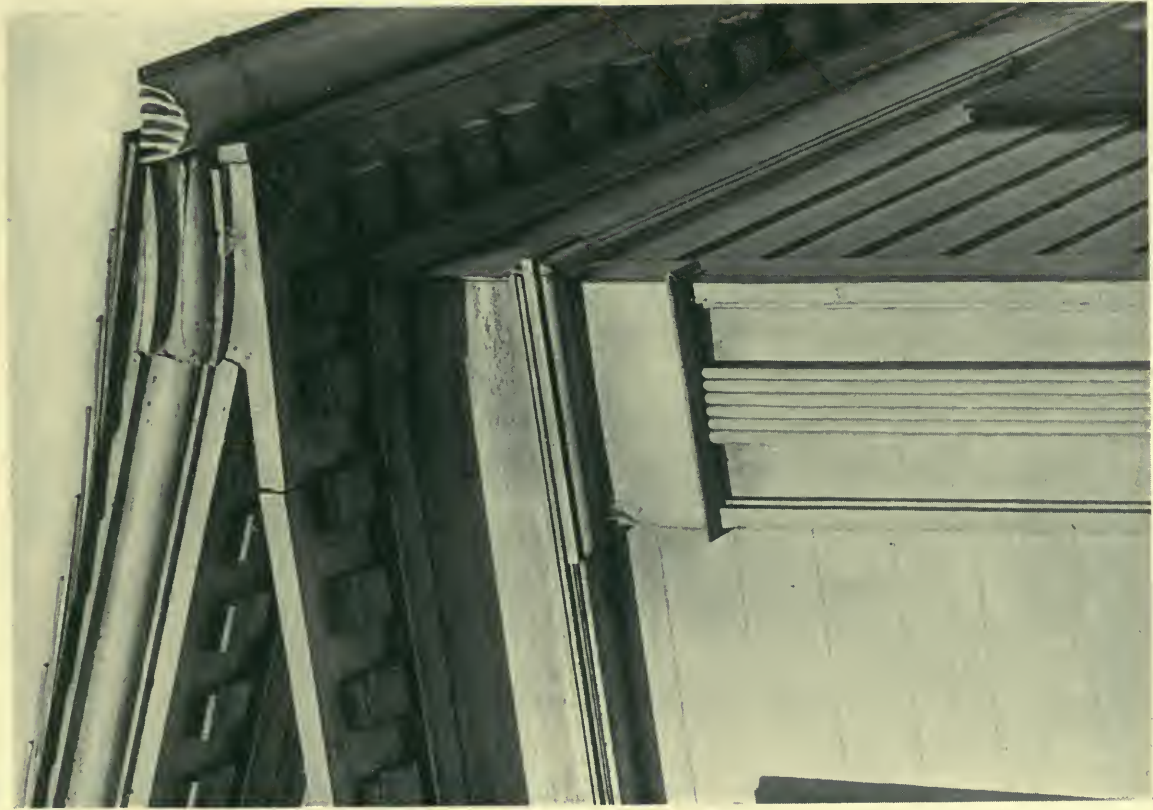
Detail of Pilaster and Pediment. DANIELS HOUSE, OWEGO, NEW YORK.
