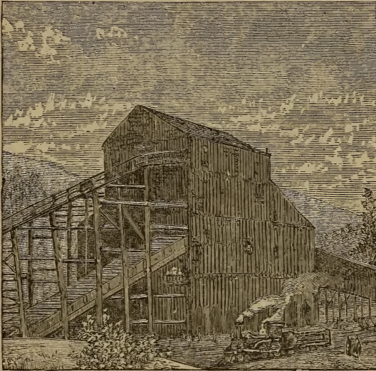
FIG. 21.— Coal-Breaker.
