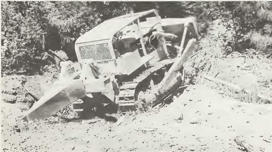
Figure 8. D9G dozer with stinger.
