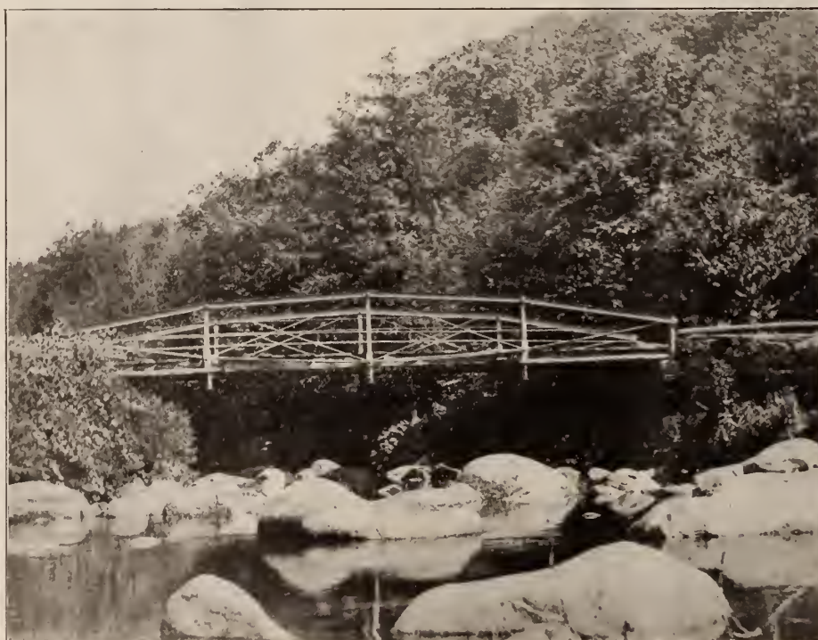
The river flowed along under the bridge carrying the red and yellow leaves
