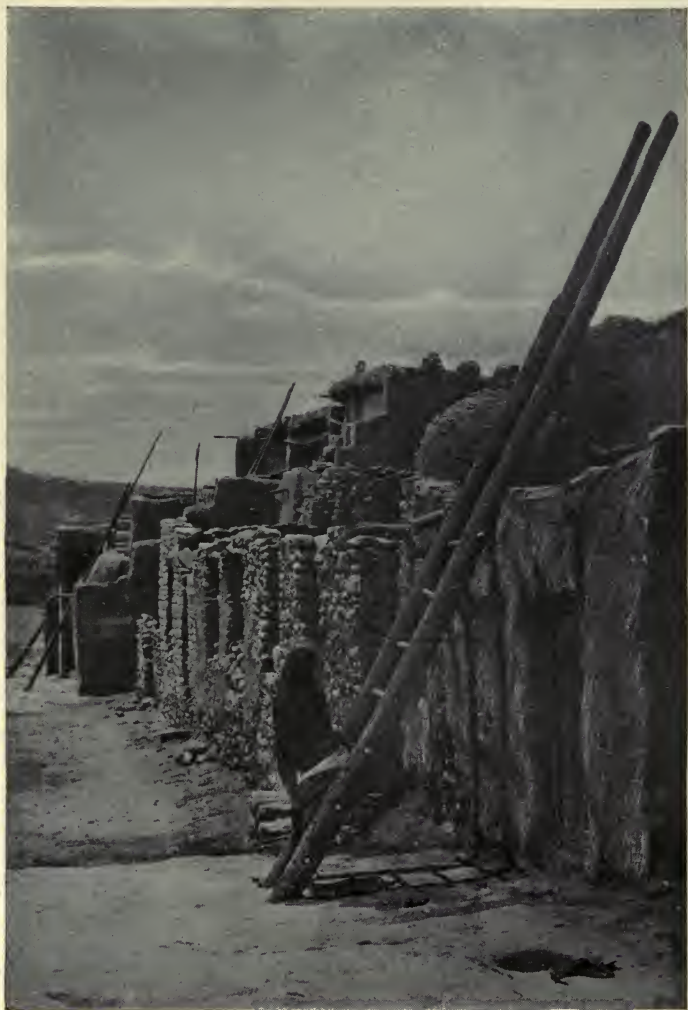
The ladders that give access to the upper stories
