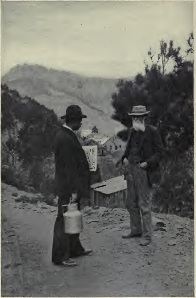
On a Black Hills roadway
