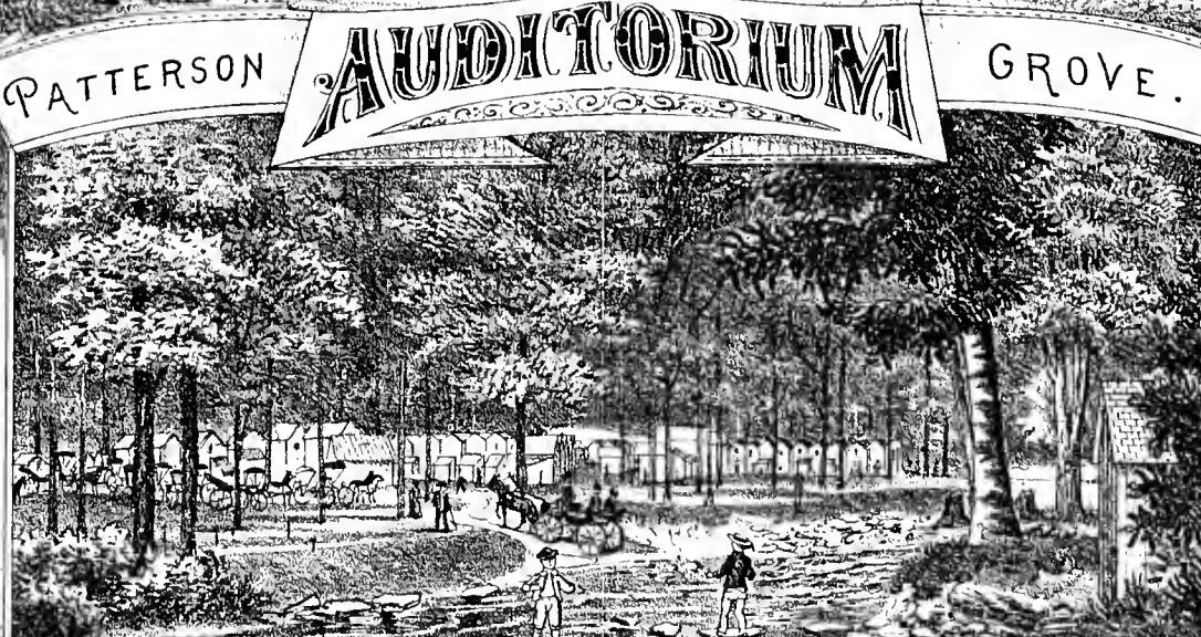
General View of the Grove and Ford over Kitchen Creek.
