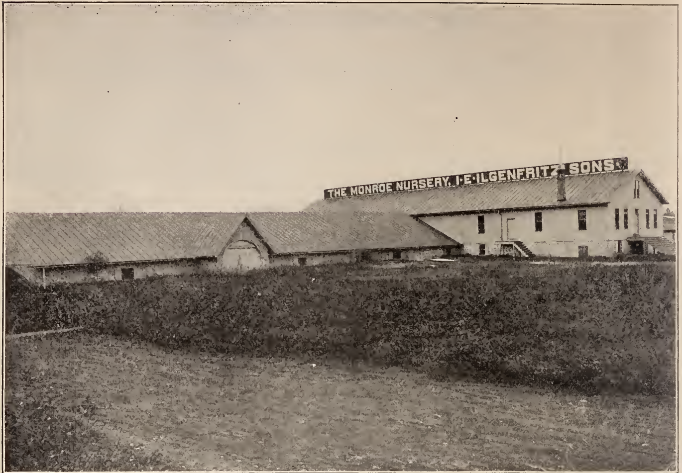
STORAGE CELLARS.—NOS. 1 AND 2.
