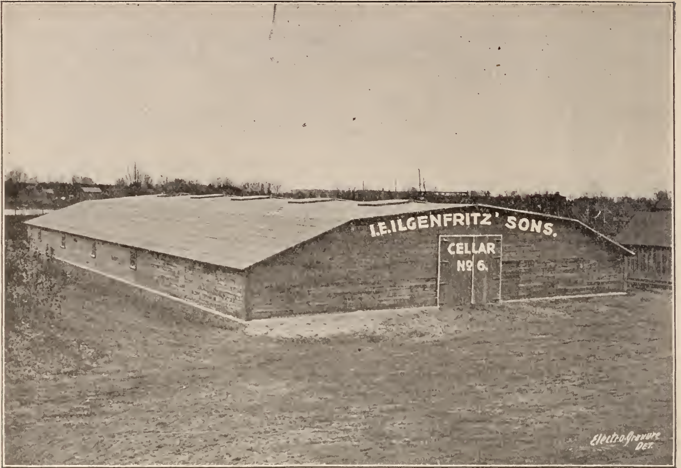
STORAGE CELLAR, NO. 6.
