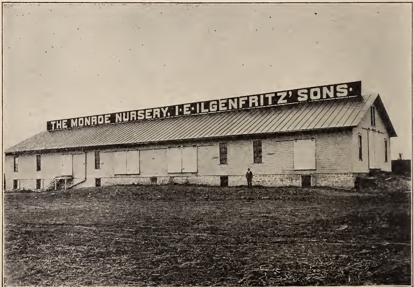
STORAGE CELLAR —NO. 2.
