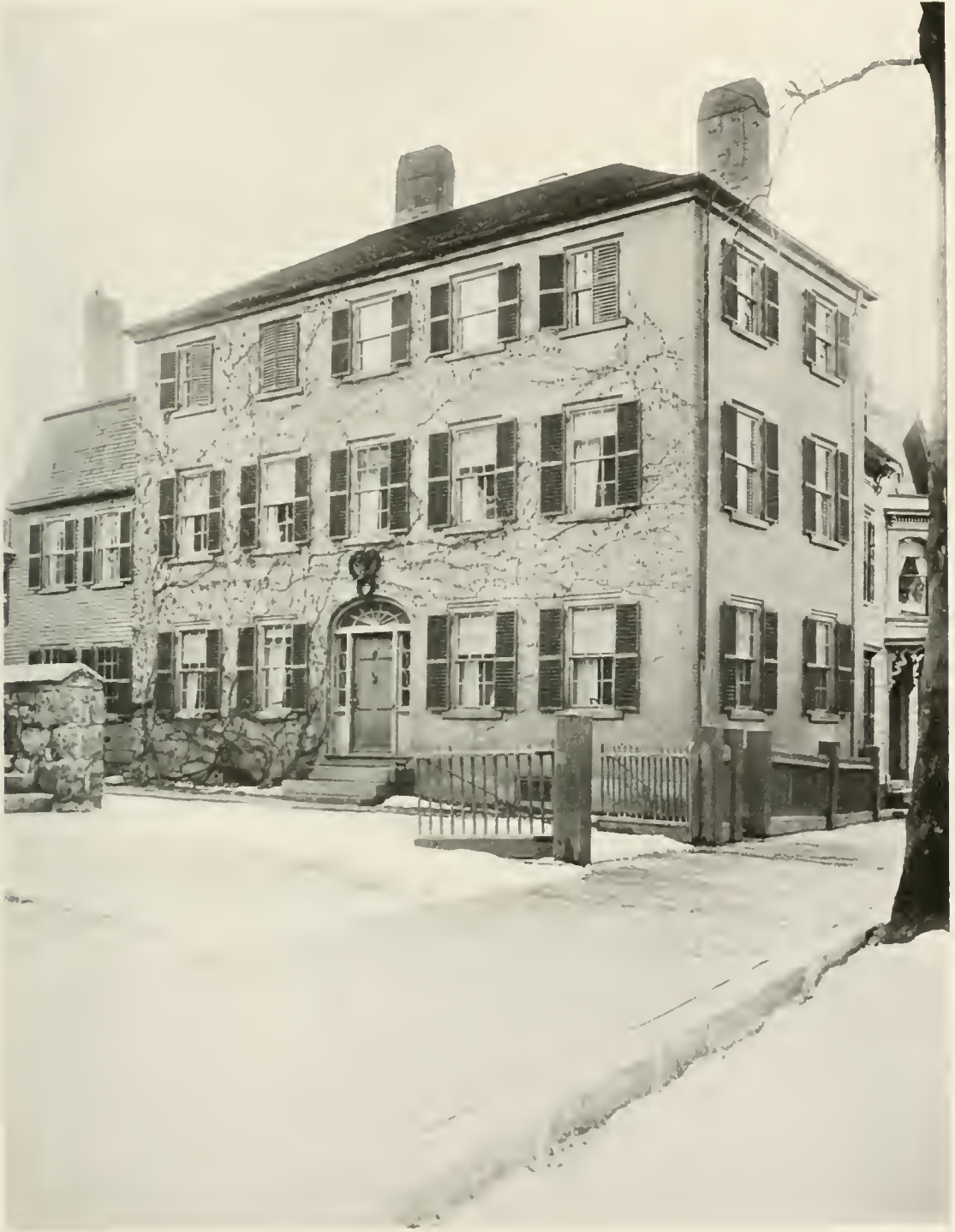
MANSFIELD-BOLLES HOUSE, SALEM, MASS BUILT ABOUT 1795
