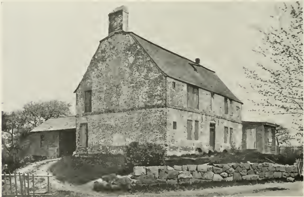
CRADOCK HOUSE, MEDFORD, MASS., BEFORE RESTORATION
