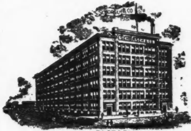
FACTORY 132 ND TO 133 RD ST & BROOK AVE
