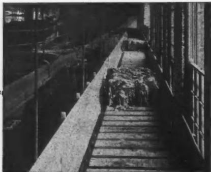
Wood Apron Conveyer Handling Bales of Rags
