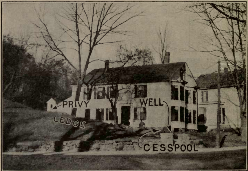
FIG. 5.—Poor relative locations of privy, cesspool, and well. (State Department of Health, Massachusetts.) Never allow privy, cesspool, or sink drainage to escape into the plot of ground from which the water supply is taken.
