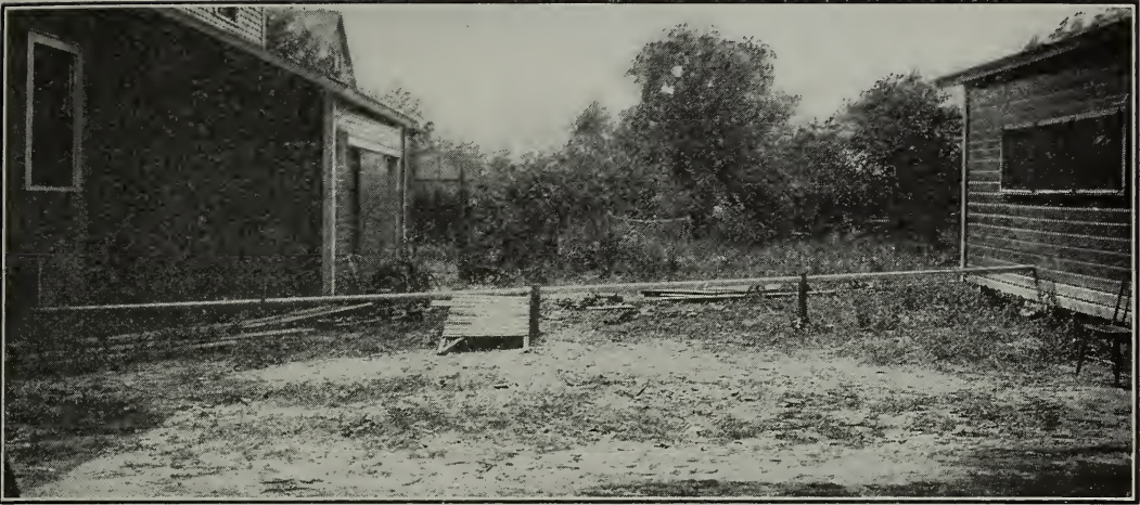
The pipe used by Chalon Fowls to convey honey from the extracting-room to the settling and straining tank in the basement of the dwelling-house.
