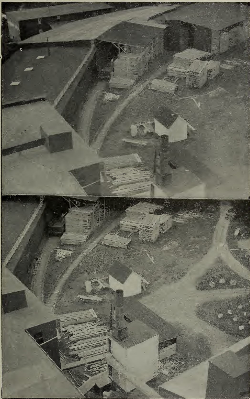
View of Covered Lumber-yard Containing the Material for Beekeepers' Supplies, as seen from the Top of the Smoke-stack.
