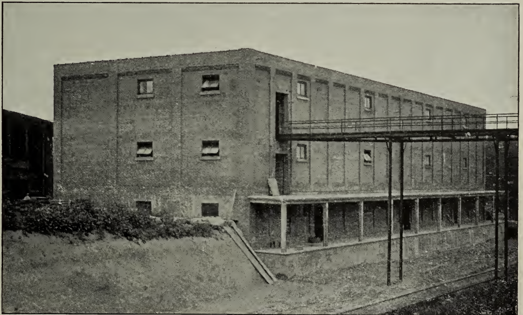
The A. I. Root Company's Fireproof Warehouse, 148 x 48, three stories, with loading-platform and steel bridge connecting old Warehouse on the south.
