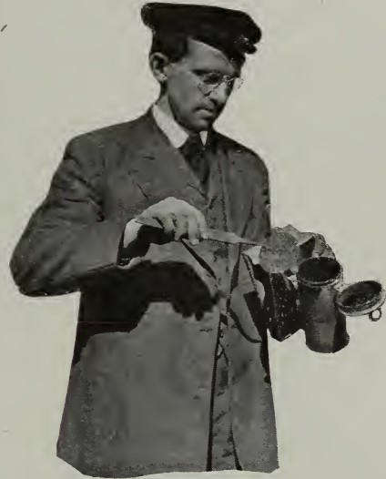
Fig. 4.—It is very seldom that a grate becomes so filled up that it has to be cleaned; but when this does happen it is the work of only a moment to insert the point of a file in one of the holes and lift out the grate, as here shown. It pays to keep the grates clean. There are a larger number of holes near the outside of the grate than in the center, consequently the fuel burns evenly and does not throw sparks until it is all consumed.
