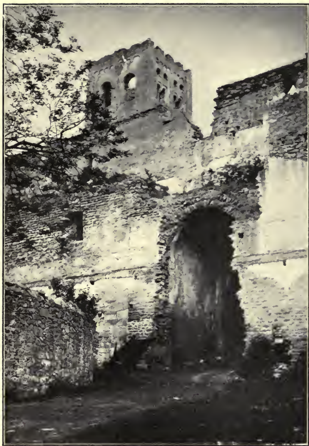
THROUGH THE BROKEN PORCH INTO THE COURT
