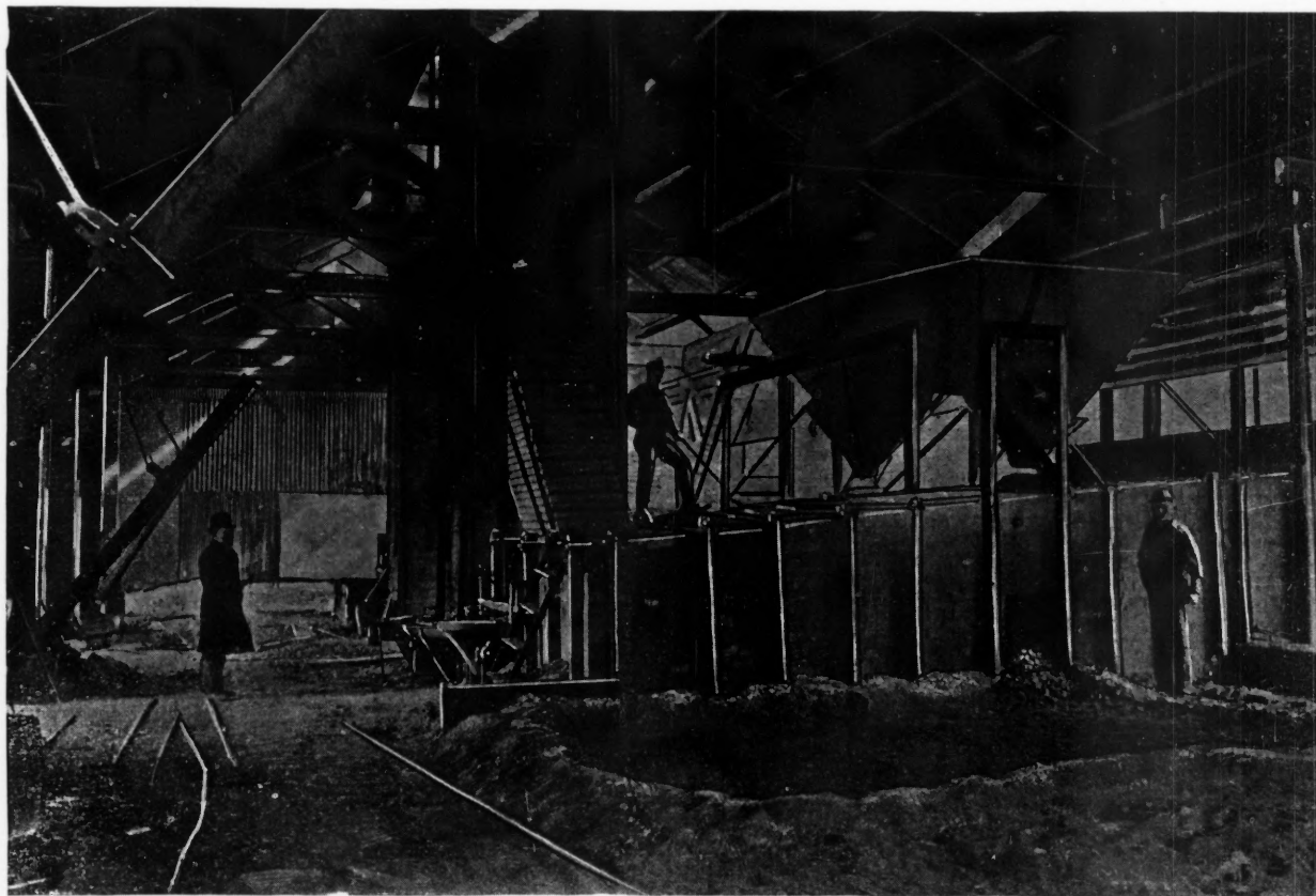
VIEW OF FURNACE FROM TAP-HOLE SIDE, AT ARGO, COLO.
