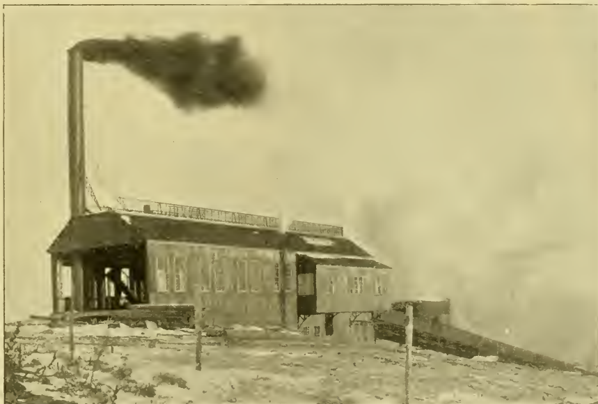
DULUTH INCLINED PLANE—POWER HOUSE.
