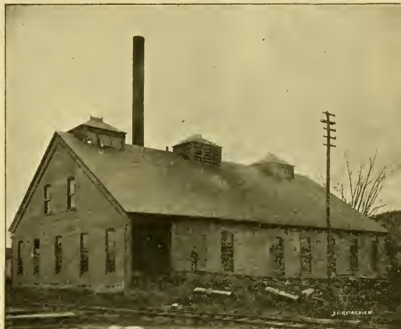
WILLIAMSPORT POWER HOUSE.
