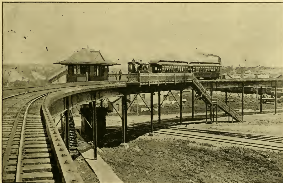
DIVISION STREET STATION ON 27 DEGREES, 10 FOOT CURVE.
