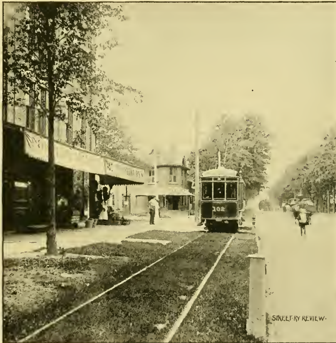
ELECTRIC LINE AT SIDE OF STREET, ROCHESTER, N. Y.
