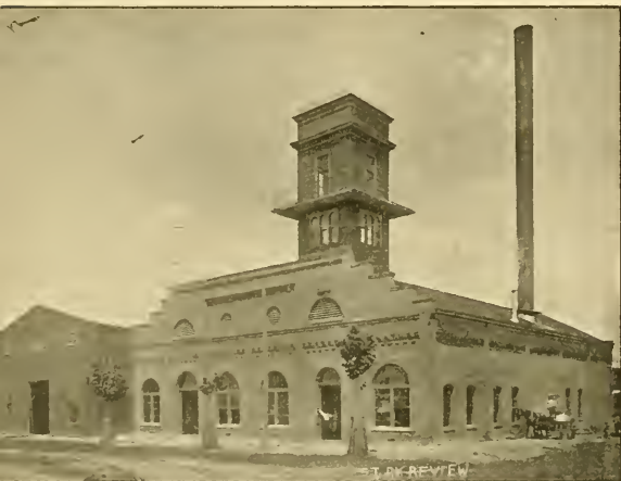
EXTERIOR OF POWER HOUSE.
