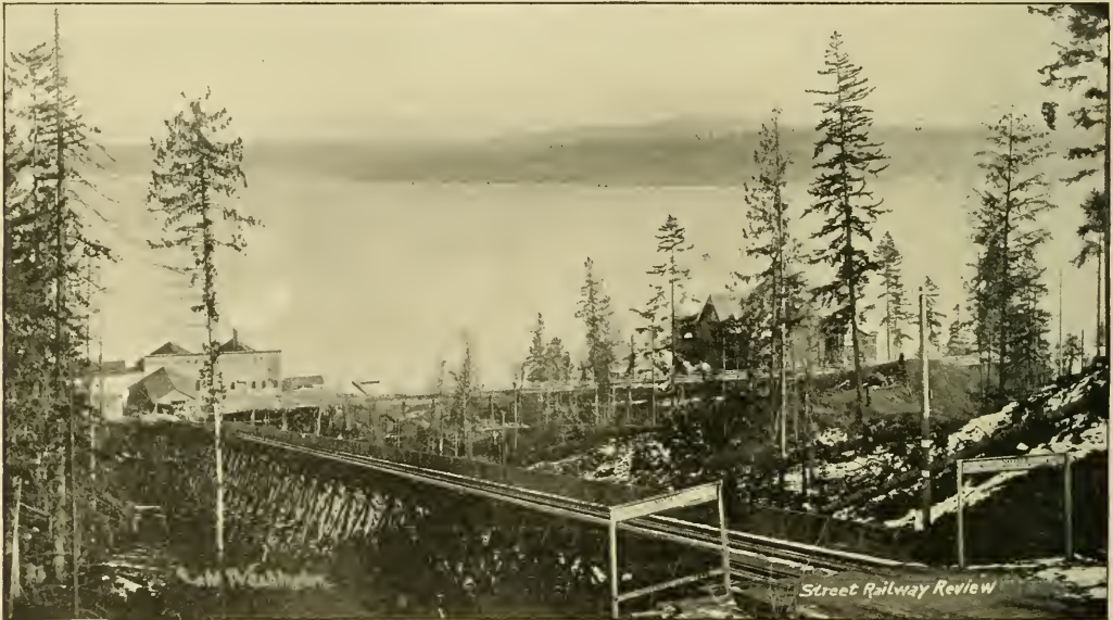
TRESTLE AT TERMINUS YESLER AVENUE CABLE LINE, SEATTLE, LOOKING TOWARD LAKE WASHINGTON.
