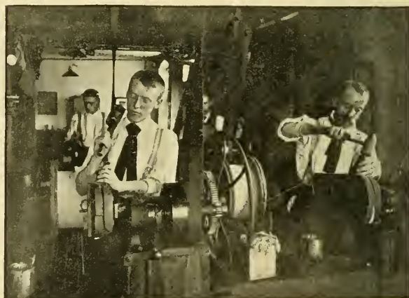
WINDING FIELD-COILS.
