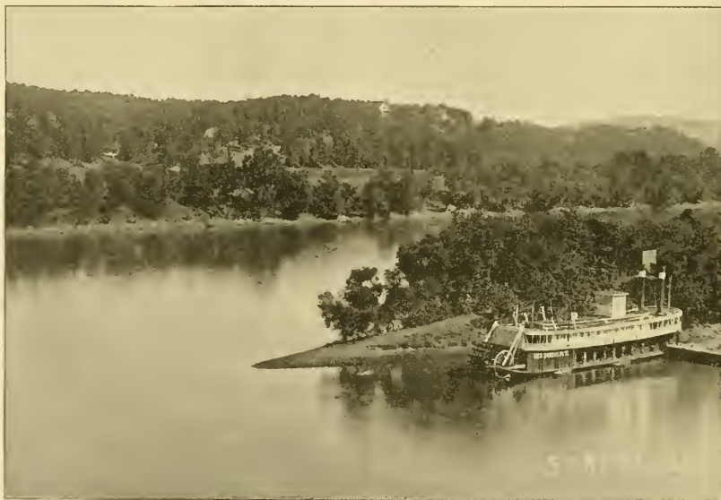
LOOKING EAST FROM THE CHATTANOOGA & NORTH SIDE RAILWAY BRIDGE.
