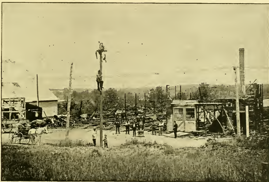
AFTER THE FIRE—NEWBURYPORT AND AMESBURY ELECTRIC RAILWAY.
