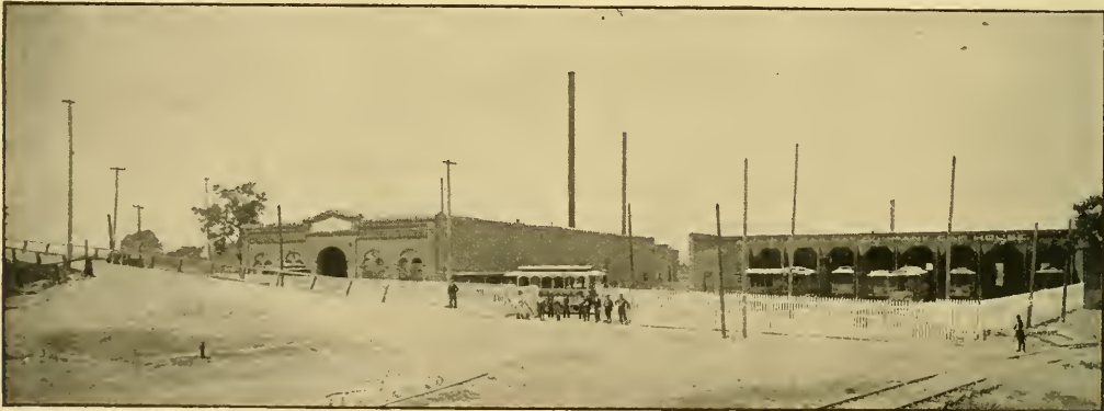
AUGUSTA ELECTRIC RAILWAY—POWER AND CAR HOUSES.
