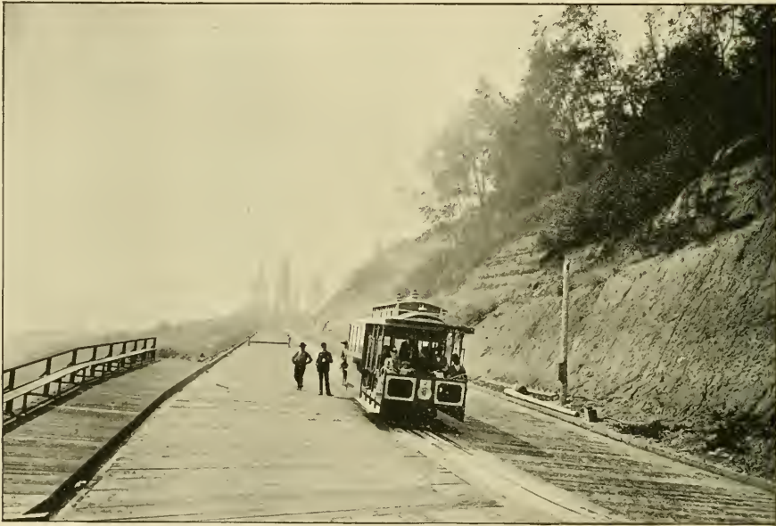
WEST SEATTLE CABLE CAR—COMING DOWN THE MOUNTAIN.
