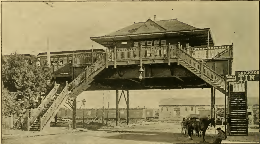
JONES STREET STATION—CITY TERMINUS.
