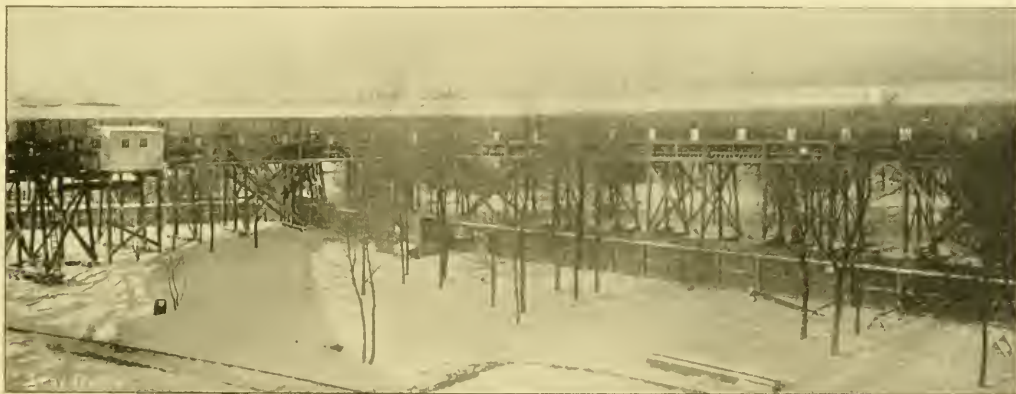
MOVABLE SIDEWALK—LOOKING NORTHWEST FROM WORLD'S FAIR GROUNDS.
