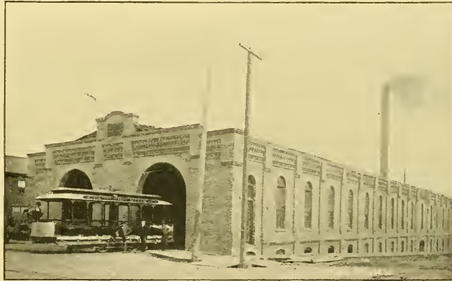
SEATTLE CONSOLIDATED RAILWAY—PINE STREET POWER HOUSE.
