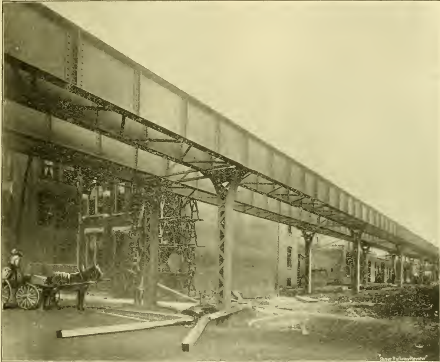
VIEW SHOWING GIRDERS AND LATERAL BRACING.
