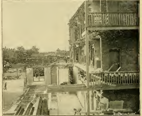
CLEARING THE RIGHT OF WAY.
