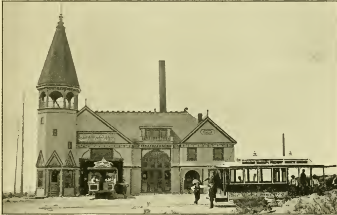
WEST SEATTLE CABLE RAILWAY POWER HOUSE.
