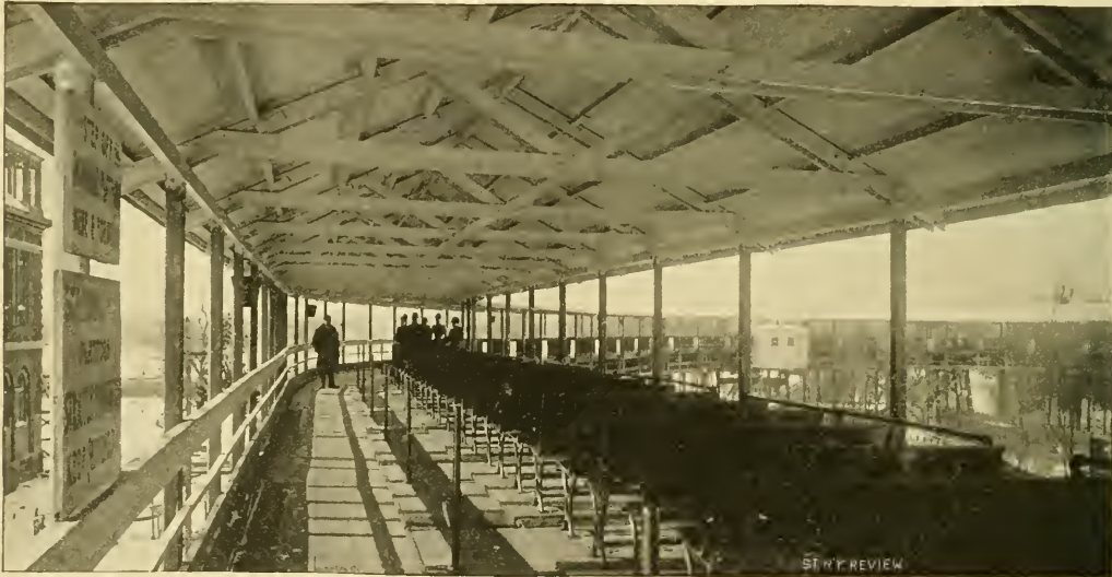
MOVABLE SIDEWALK—PLATFORMS AND SEATS.
