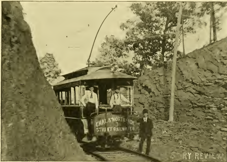
THROUGH A HILL ON THE CHATTANOOGA & NORTH SIDE RAILWAY.
