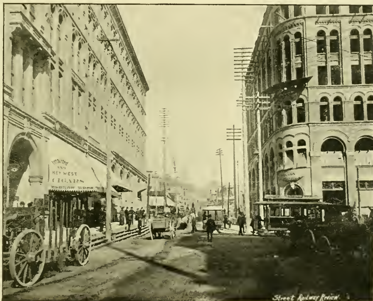
TURN TABLE AT FOOT YESLER AVENUE, CABLE, SEATTLE.
