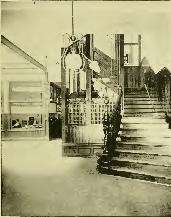
CHICAGO CITY RAILWAY BUILDING—MAIN ENTRANCE.
