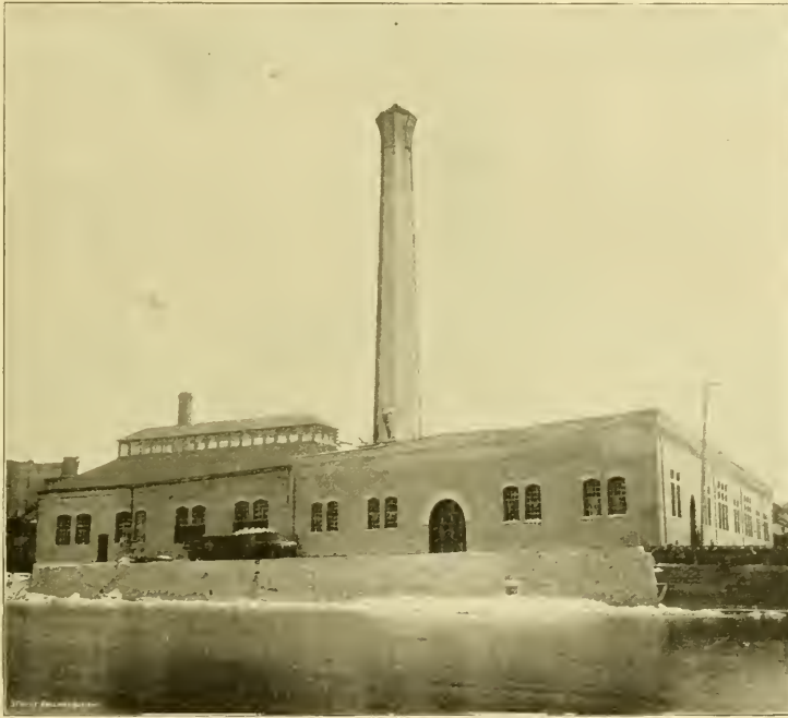
POWER HOUSE AS SEEN FROM OPPOSITE BANK OF FOX RIVER.
