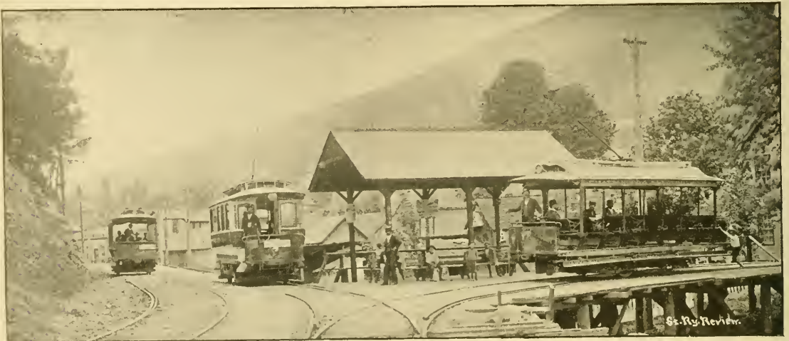
LOOKOUT MOUNTAIN INCLINE JUNCTION.
