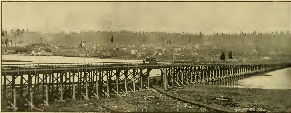
BRIDGE 6,000 FEET IN LENGTH, OVER THE FLATS, FOR THE WEST STREET AND NORTH END ELECTRIC LINE.
