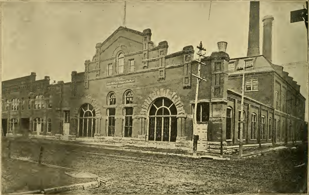
MAIN POWER STATION, BROADWAY CABLE LINE, ST. LOUIS.
