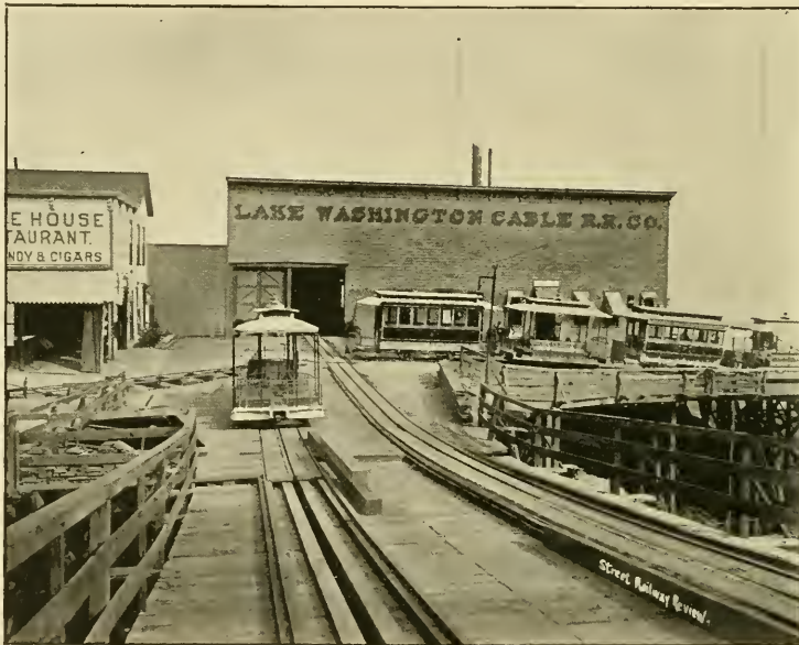
POWER HOUSE, YESLER AVENUE CABLE LINE, SEATTLE.
