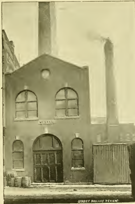
POWER HOUSE 25 FEET WIDE.
