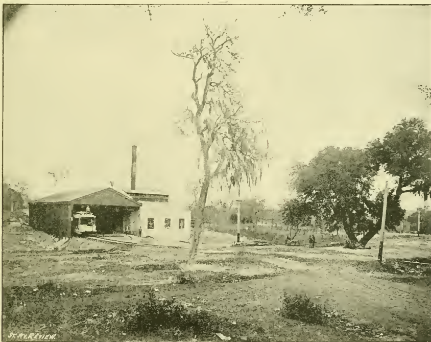
POWER HOUSE SAN ANTONIO ELECTRIC RAILWAY.
