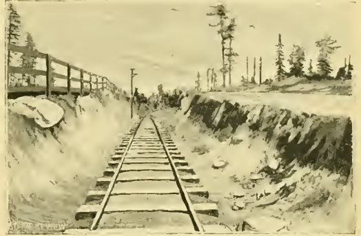
A LONG CUT ON GRADE.
