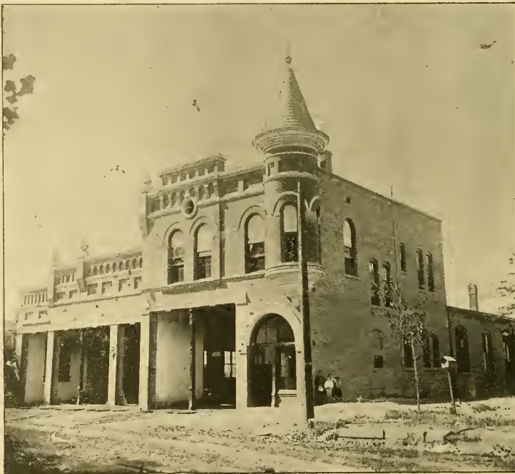
FRONT VIEW ON TRACK LEVEL, OF LITTLE ROCK POWER HOUSE.
