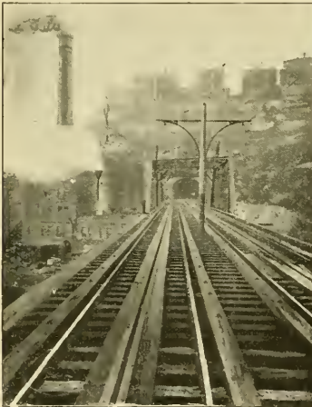
POWER HOUSE AT WEST END OF TUNNEL.
