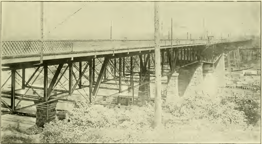
SUPERIOR STREET VIADUCT.
