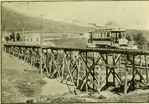
TRESTLE ON THE SAN MATEO LINE.
