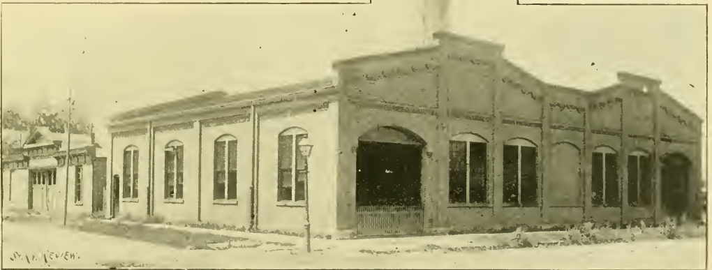
POWER HOUSE—BROOKLYN STREET RAILROAD—CLEVELAND.
