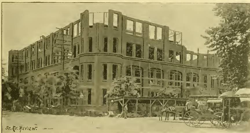
POWER HOUSE AS IN PRESENT COURSE OF CONSTRUCTION.
