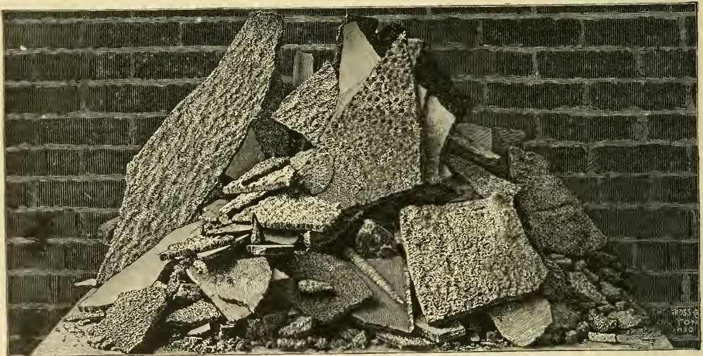
LIME DEPOSITS REMOVED FROM WATER PURIFIER AT DAYTON (OHIO) CITY WATER WORKS.
