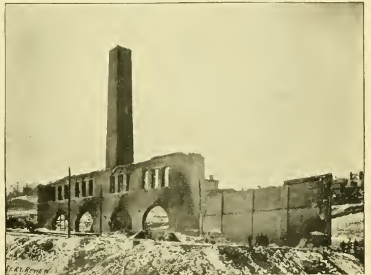
RUINS MT. AUBURN CABLE POWER HOUSE.
