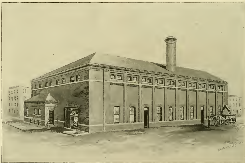
THE BOILER HOUSE.
