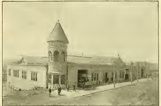
SAN MATEO POWER STATION.
