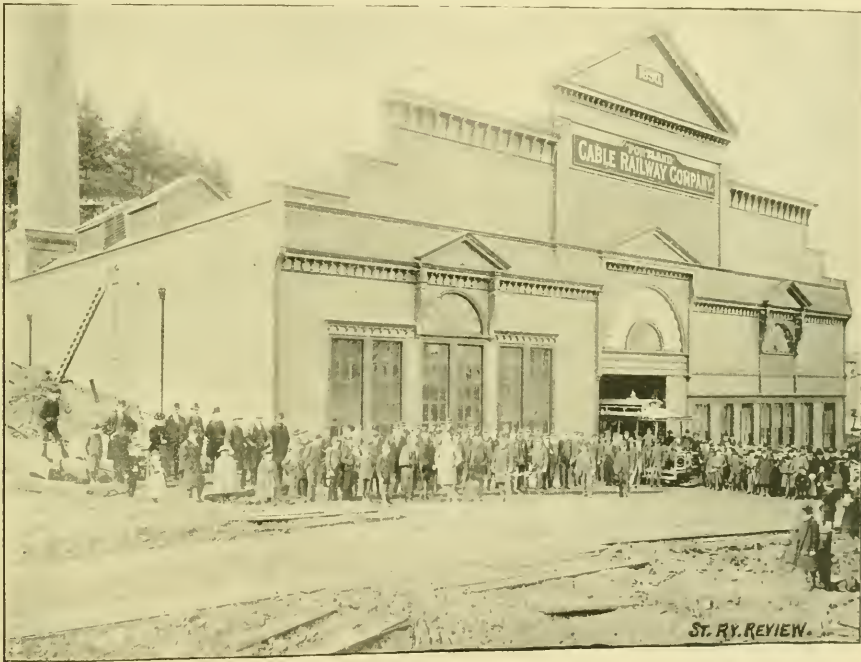
POWER HOUSE PORTLAND CABLE RAILWAY.
