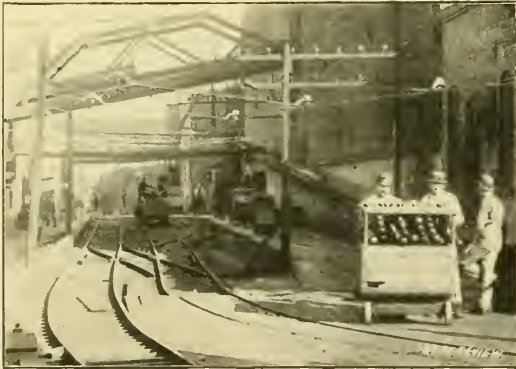
FLOOR OF ELEVATED STRUCTURE—41ST ST. AND PACKER'S AVE.
