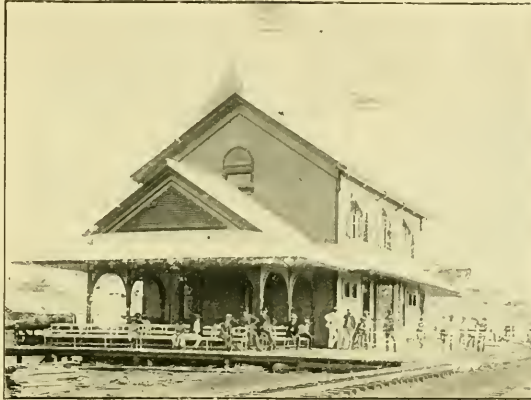
STEAM RAILROAD STATION, HONOLULU, S. I.
