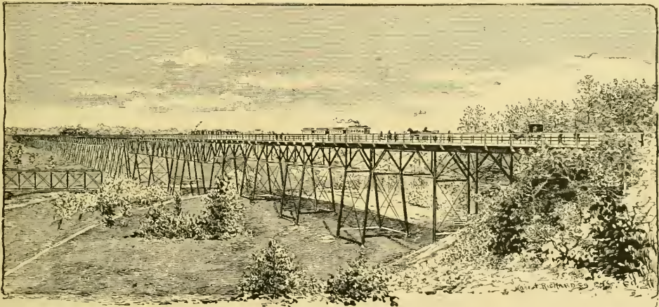
VIADUCT OVER THE MENOMINEE VALLEY.
