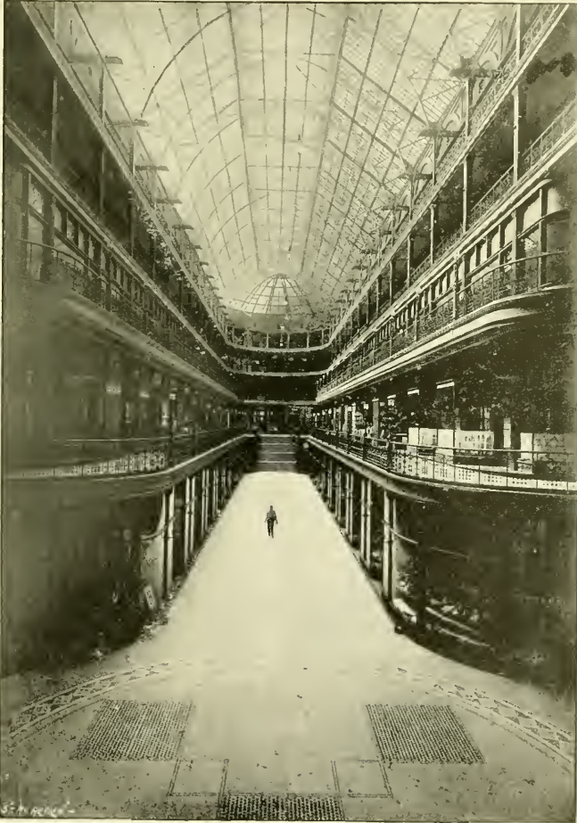
INTERIOR OF THE ARCADE BUILDING.
