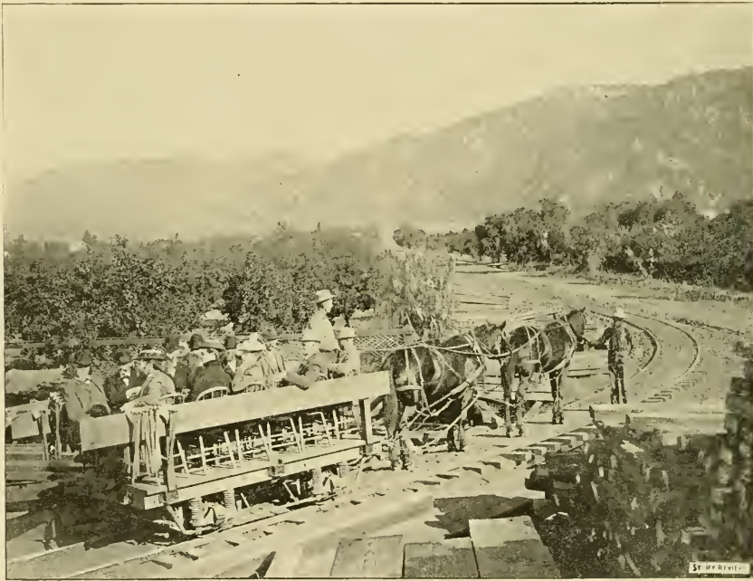
TEMPORARY TRANSPORTATION DURING CONSTRUCTION.
