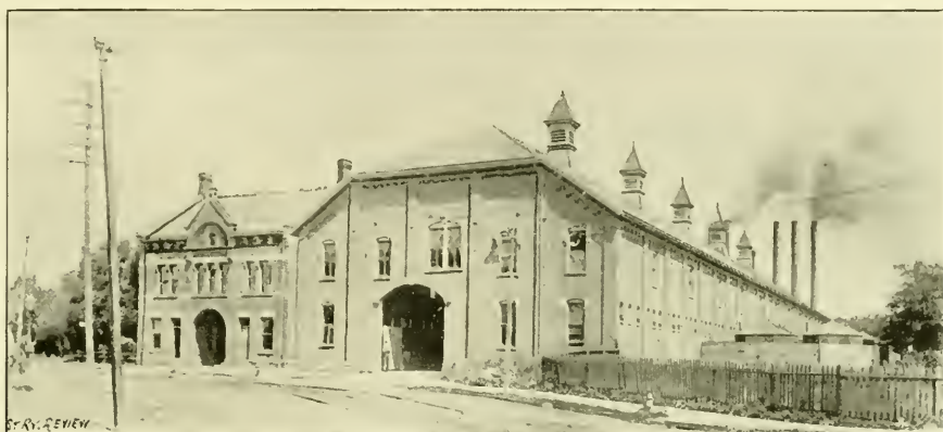
POWER HOUSE—BROADWAY AND NEWBURG.
