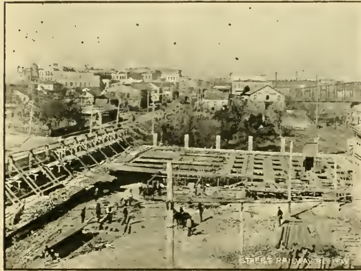
CAR HOUSE UNDER CONSTRUCTION.
