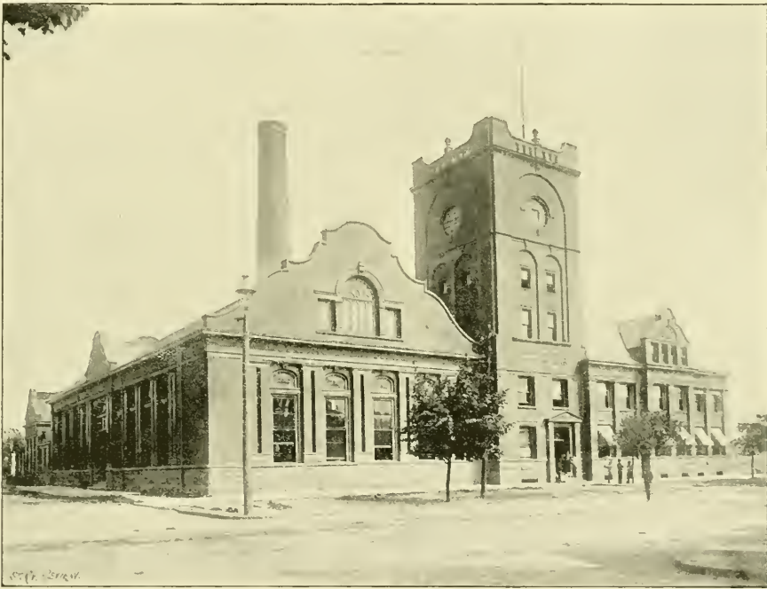
CLEVELAND CITY CABLE POWER HOUSE.
