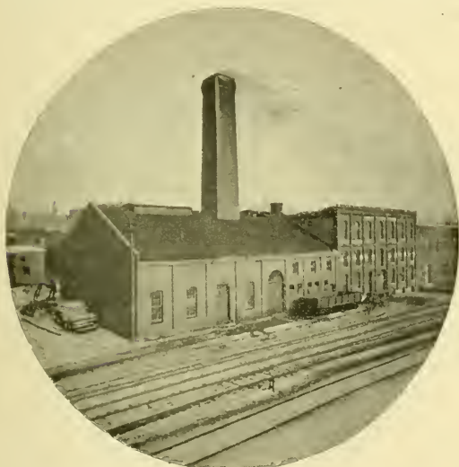
THE POWER PLANT.
