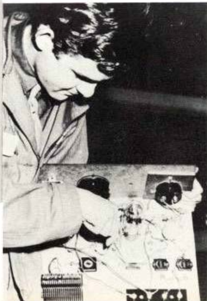
Bread-board receiver design in the Radio Fundamentals Branch.
