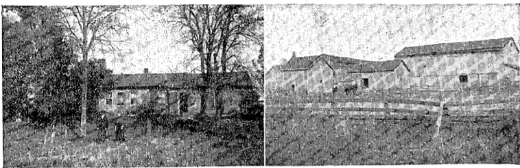
RESIDENCE AND FARM BUILDINGS OF E. A. BREWSTER.
