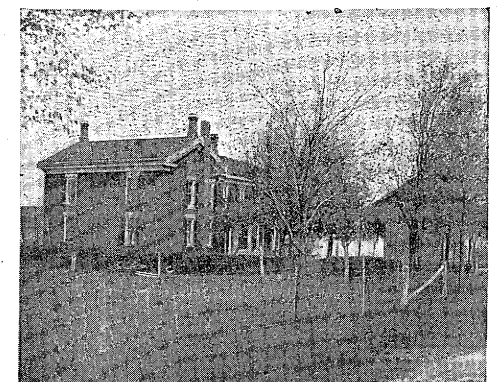
RESIDENCE AND FARM BUILDINGS OF A. D. DE GARMO.
