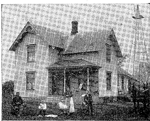
RESIDENCE OF PETER ADDIS.
