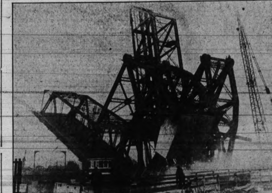
The Bridge Open, During Construction
