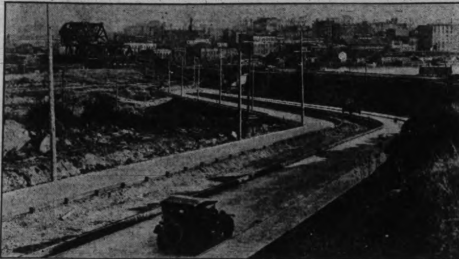
The New Roadway, Looking East From the Rock Cut
