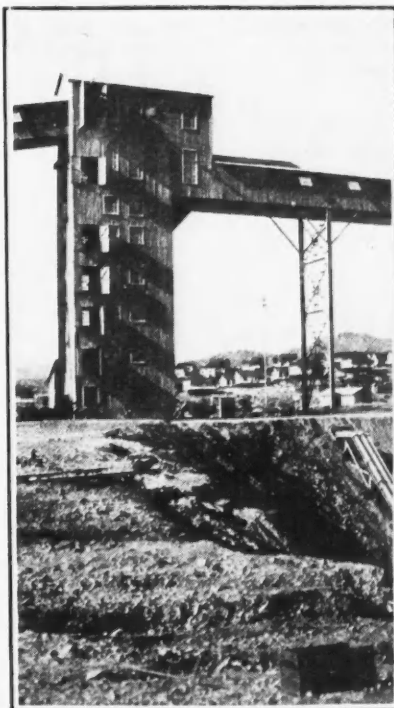
Sampling plant of the Miami mill at Miami, Ariz.
