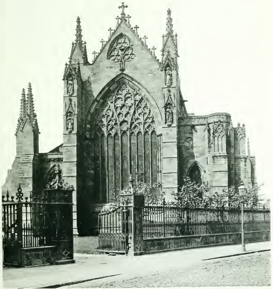
CARLISLE CATHEDRAL, EAST FRONT.
