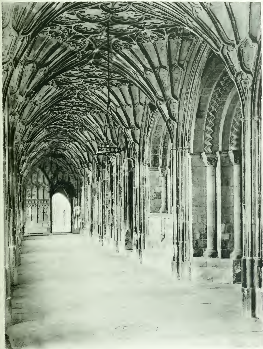
GLOUCESTER CATHEDRAL, THE CLOISTERS.
