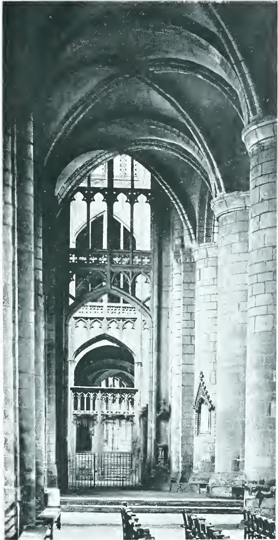
Gloucester, North Aisle of Nave.
