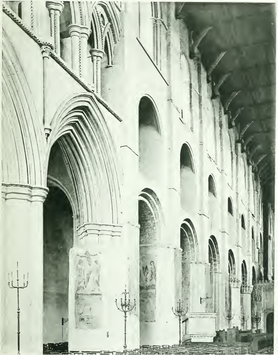
ST. ALBANS, NAVE FROM S.W.
