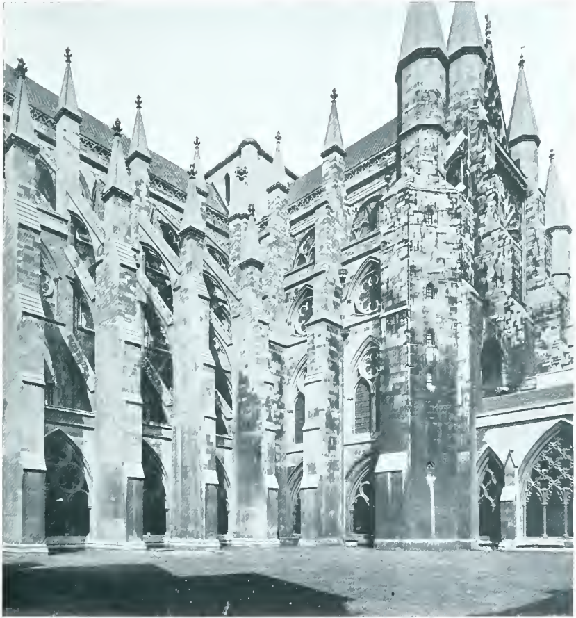
Westminster Nave and South Transept.
