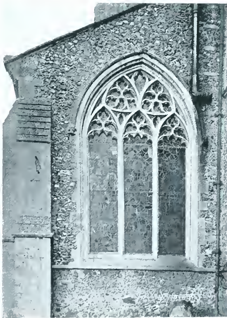
Westminster Cloister. Hingham S. Aisle.
