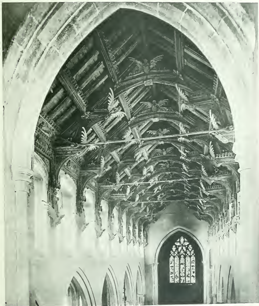
MARCH, ROOF OF NAVE.
