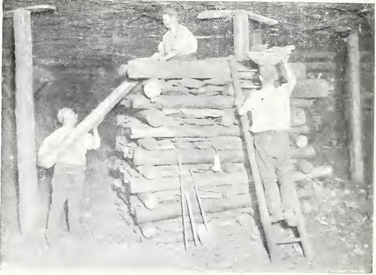
Building a Timber Cog.—HERBERT W. HUGHES.
