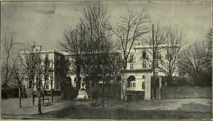
The School seen from the Road.
