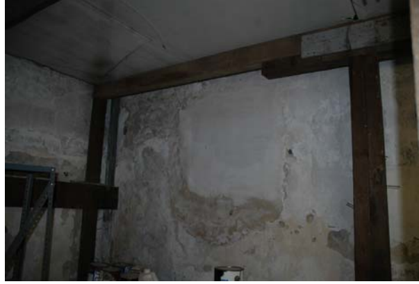
Figure 1.5-39: Detail view of plaster damage (left) and plaster patches (right) in Room 115.
