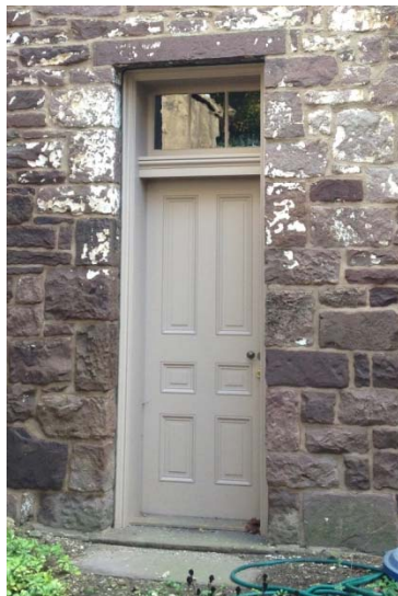
Figure 1.5-11: (Left) The door in the west elevation opening to the courtyard is in good condition. Its age is yet to be determined. (Right) The door in the south elevation exhibits minor to moderate paint failure in scattered locations but otherwise appears to be in good condition.
