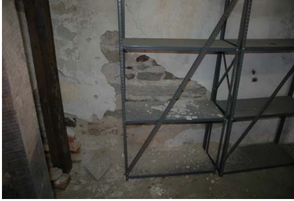
Figure 1.5-39: Detail view of plaster damage (left) and plaster patches (right) in Room 115.
