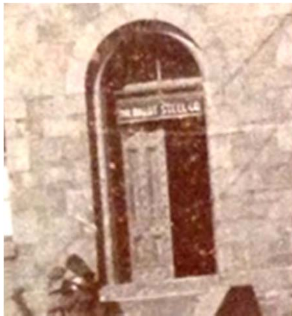
Figure 1.2-9: Detail of the above photograph dated c. 1903. The name Baldt Steel Company is painted on the transom of the front door.
