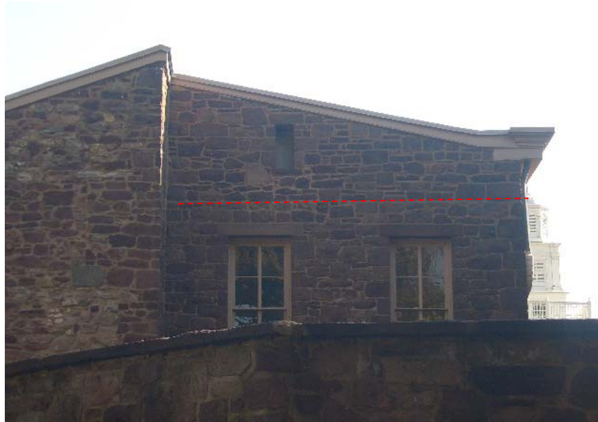
Figure 1.2-30: A masonry seam above second-story windows suggests that the west wall preceded the 1857 construction and was raised as the north end became part of the prison tower.
