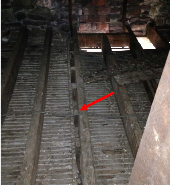
Figure 1.2-41: The framing for the north-south partition separating 207 and 208 is much smaller in dimension than the partitions dividing the center hall and is likely a different vintage.
