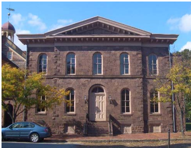
Figure 1.3-12: The arched windows on the east façade, characteristic of the Italianate style, reflect the hierarchy of the interior floors. The windows on the first floor are tallest while those on the second story, though similar in shape, are slightly shorter. The basement windows are smallest.
