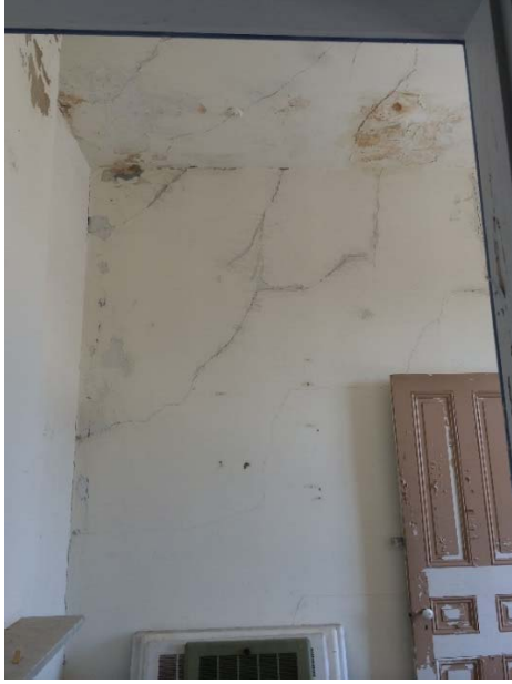
Figure 1.5-40: South view of wall and ceiling plaster cracking and water damage in Room 201 (left) Detail view of water damage at window head in Room 201 (right).
