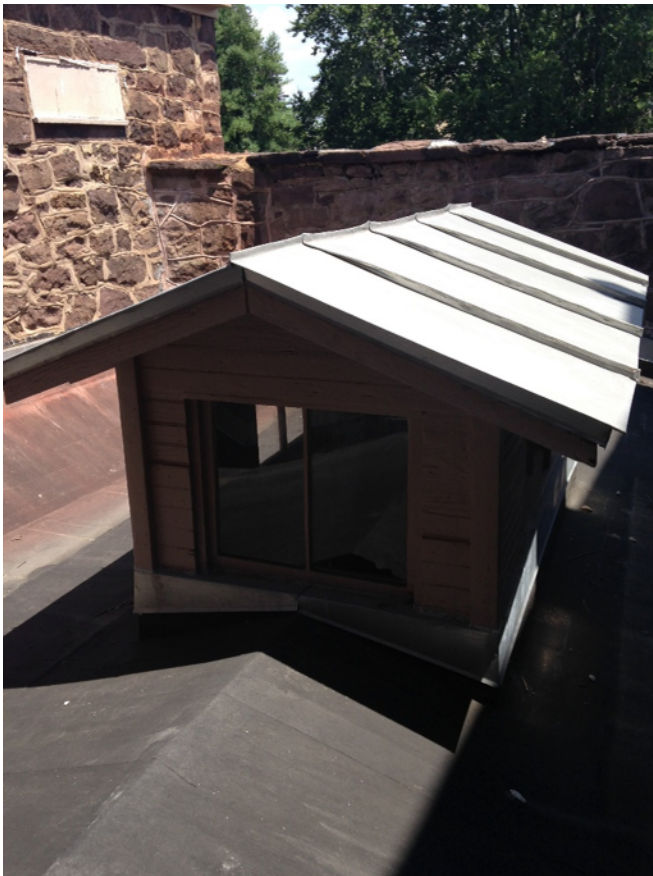
Figure 1.3-6: Roof plan. Note the multiple intersecting slopes resulting from the intersection of the Sheriff's House with the surviving portion of the prison.
