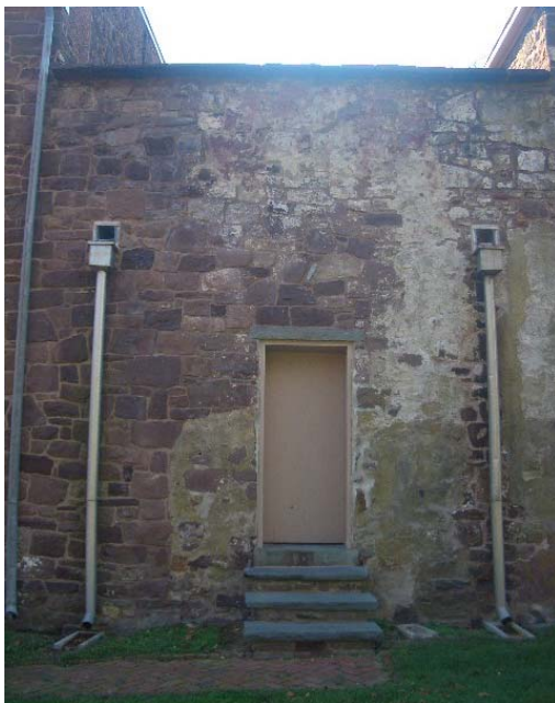
Figure 1.2-15: (Left) The wall at the center of the north elevation formed an original open courtyard. The scuppers mark the level of the roof that was later constructed to cover the courtyard. The existing door opening appears in the 1911 photograph of the prison demolition (Right).
