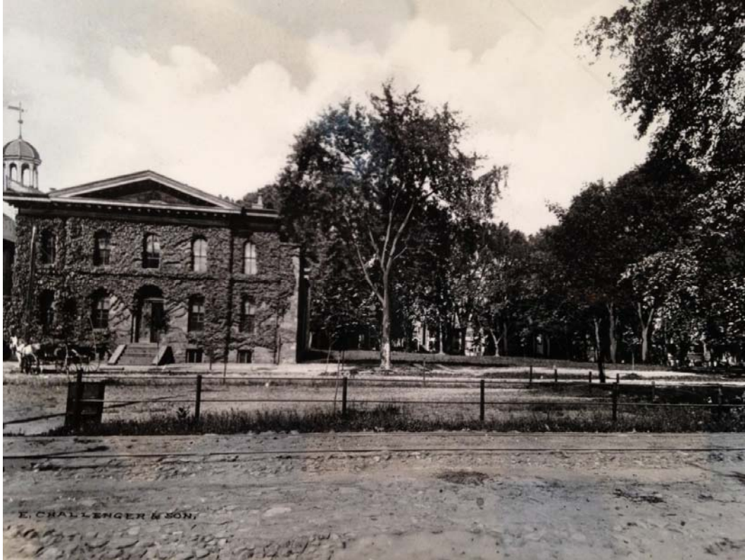
Figure 1.2-10: Photograph of the Sheriff's House c. 1911. Note that the jail and its surrounding walls have been demolished. The building also seems somewhat unkempt as evidenced by the ivy spreading across the entire facade. 48
