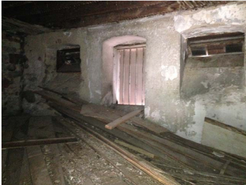
Figure 1.2-43: East wall of Room 210. This room is shown on the insurance maps as two cells and the two narrow horizontal windows are consistent with that assumption. However, the dividing wall has been removed to form a single large room. The walls have been replastered and an additional window installed. This change occurred prior to the closing of the prison.
