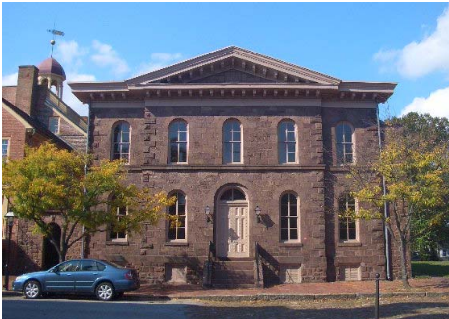
Figure 1.1-9: East elevation of the New Castle Sheriff's House. Note the similarities between this façade and those from City and Suburban Architecture shown in Figure 1.1-8 above. Photograph by John Milner Architects, Inc., October 2015.
