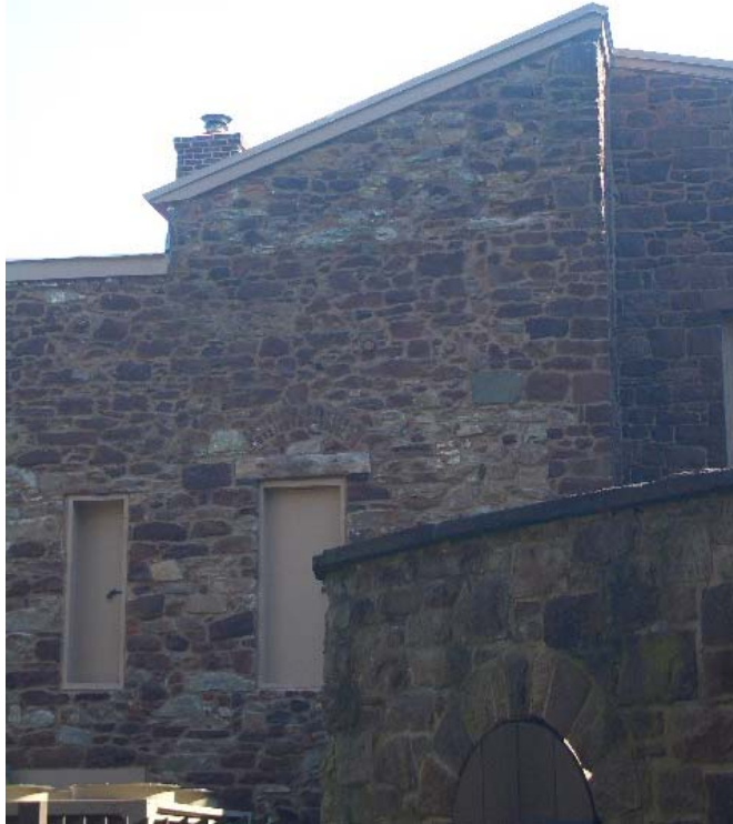
Figure 1.2-64: Openings in the west wall masonry correspond to the entrances to the remaining cells. The brick arch of the opening on the right indicates an original cell door. The narrower door on the left opens into a single large room that may have been formed when two cells were combined.
