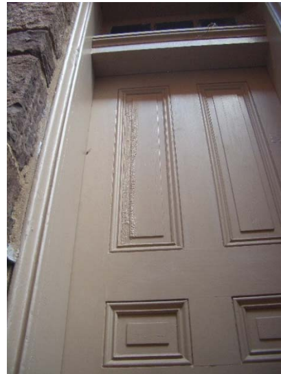
Figure 1.5-11: (Left) The door in the west elevation opening to the courtyard is in good condition. Its age is yet to be determined. (Right) The door in the south elevation exhibits minor to moderate paint failure in scattered locations but otherwise appears to be in good condition.
