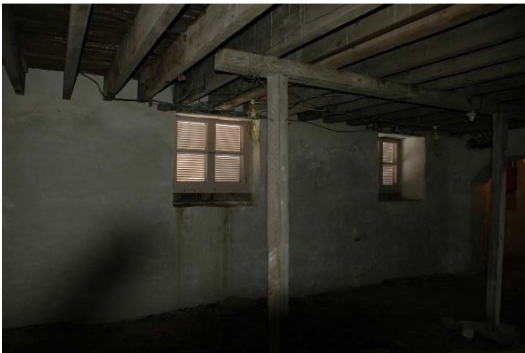
Figure 1.3-16: Views of Room 001 looking northwest (top) and looking southeast (bottom).
