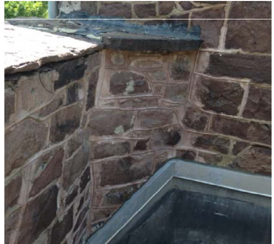
Figure 1.2-14: (Left) First-floor plan of the Sheriff's House. The room adjoining the north parlor was once an exterior yard. (Right) The interior corners have been infilled with masonry to prevent prisoners from climbing out.
