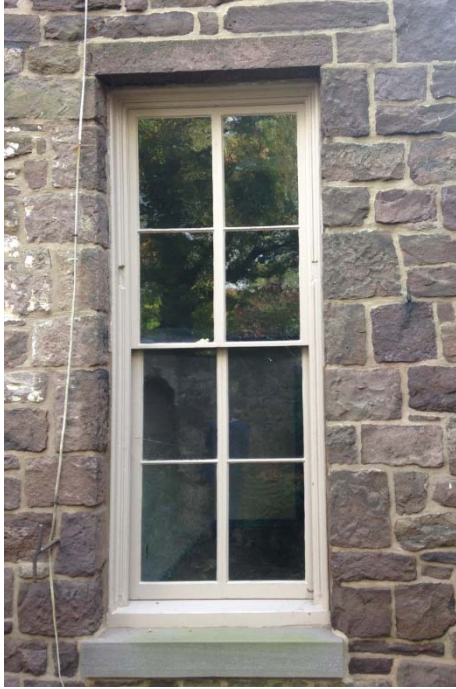
Figure 1.5-15: (Left) The windows on the south and west facades are of similar muntin configuration as those on the front of the building. The sills and sashes also appear to be replacements. (Right) The basement windows and their louvered shutters are in very good condition aside from minor to moderate soiling.
