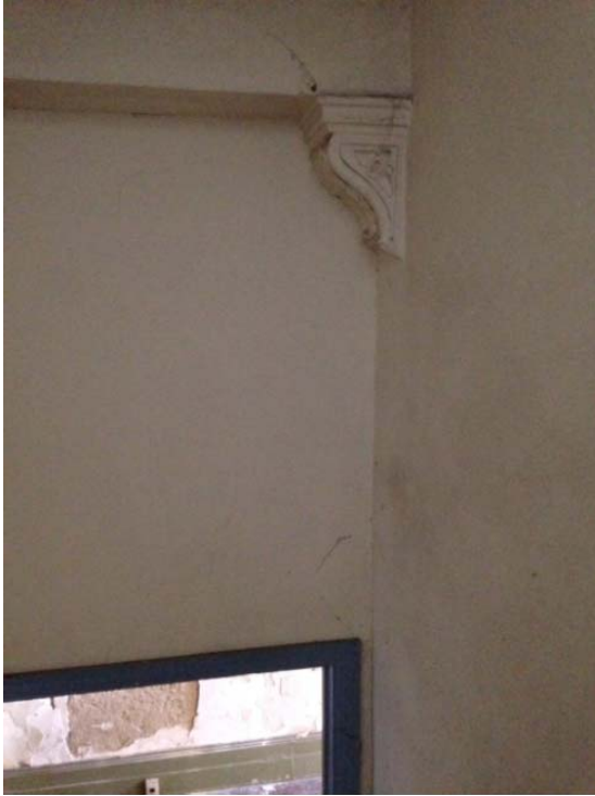
Figure 1.2.71: (Left) The modern partition blocks the opening to the stair hall, concealing the decorative brackets. (Right) Another stud and drywall partition encloses the side of the stair as well.
