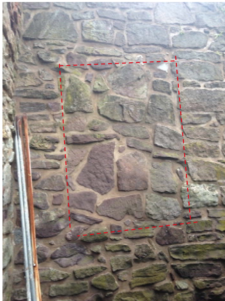
Figure 1.2-32: (Upper Right) A line of mastic above the west door and traces of whitewash around the door opening define the dimensions of a former structure. Whether this was a connector to the prison as shown on the 1885 plan or simply a later porch has not been determined. (Upper Left) The mastic line continues around onto the courtyard wall. (Lower Left) A closed window opening is visible in the north side of the courtyard wall.
