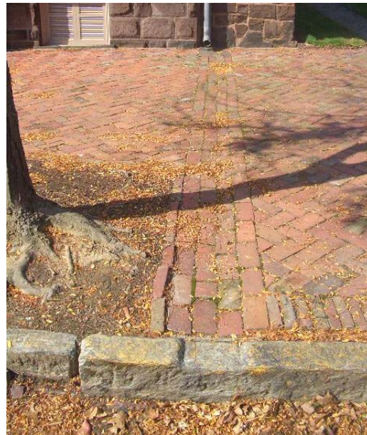
Figure 1.5-3: (Left) The brick-paved walking surface in front of the Sheriff's House is in good condition despite settlement of individual bricks. The surface is generally level with minor lipping. (Right) Tree roots have dislodged bricks in their immediate vicinity as well as some curb stones.
