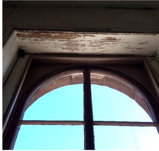
Figure 1.5-40: South view of wall and ceiling plaster cracking and water damage in Room 201 (left) Detail view of water damage at window head in Room 201 (right).
