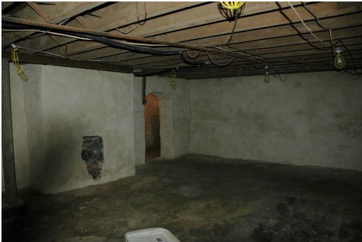
Figure 1.3-21: Views of Room 006 looking southwest (top) and looking northeast (bottom).
