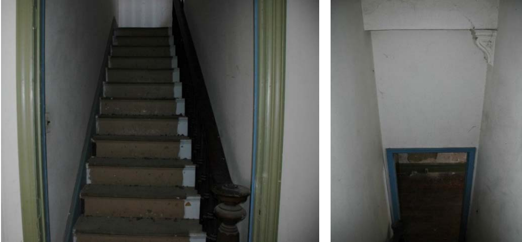
Figure 1.3-25: Views of Room 104 looking south up the main stair to the second floor (left) and looking north with an original plaster bracket visible (right).
