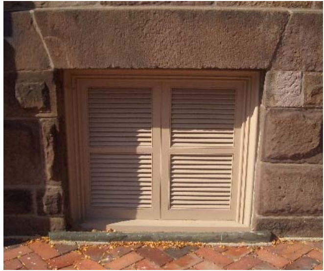
Figure 1.5-15: (Left) The windows on the south and west facades are of similar muntin configuration as those on the front of the building. The sills and sashes also appear to be replacements. (Right) The basement windows and their louvered shutters are in very good condition aside from minor to moderate soiling.
