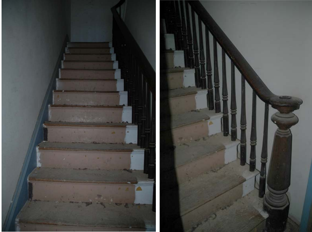
Figure 1.5-27: Views of the wood stair in Room 104.
