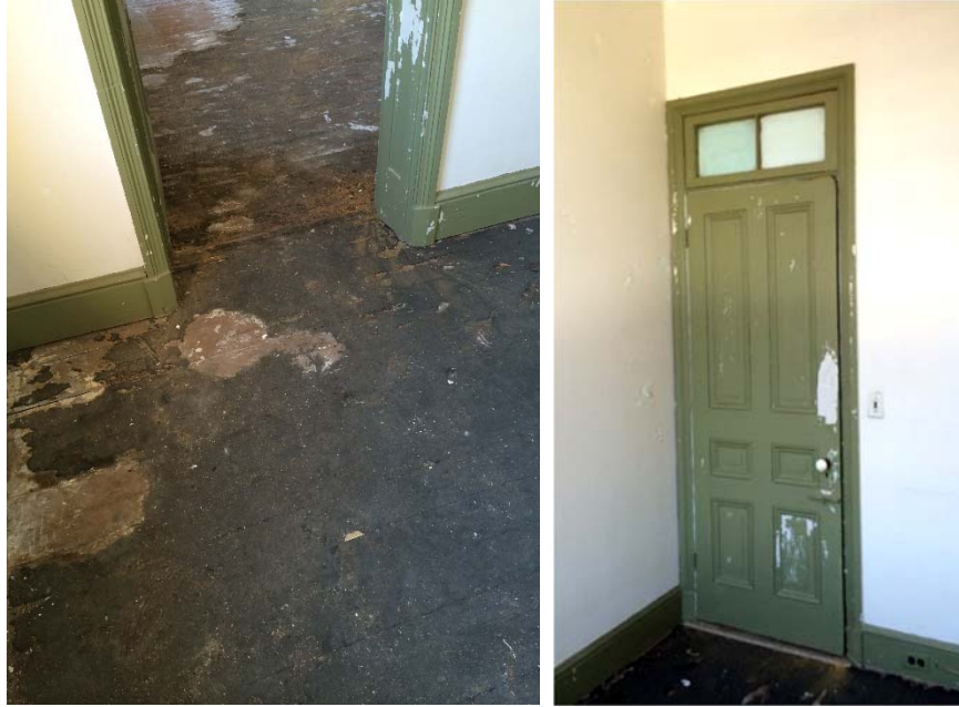
Figure 1.5-43: Detail view of modern flooring remnant over original floor in Room 204 (left). Detail view of west door and transom in Room 204 (right).
