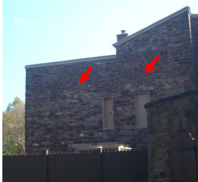
Figure 1.2-44: Room 210 shown on the existing second-story plan (left) consists of approximately 2½ upper tier cells. The door to the south cell remains intact with its relieving arch (right arrow) while only traces of the relieving arch remain of the door to the north cell (left arrow).
