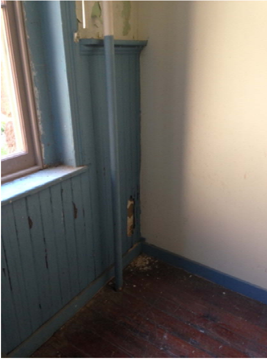
Figure 1.2-61: (Left) Wainscot was installed over the original wall plaster in the southwest kitchen c. 1915-1920. (Right) This fireplace was likely built c. 1920 after the original fireplace on the south wall was removed.
