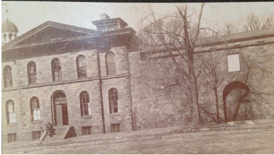
Figure 1.2-8: Photograph of the Sheriff's House c. 1903. The name Baldt Steel Company is painted on the transom of the front door. Note the prison tower still standing in the background and the presence of what appear to be interior shutters on all of the visible windows. 38
