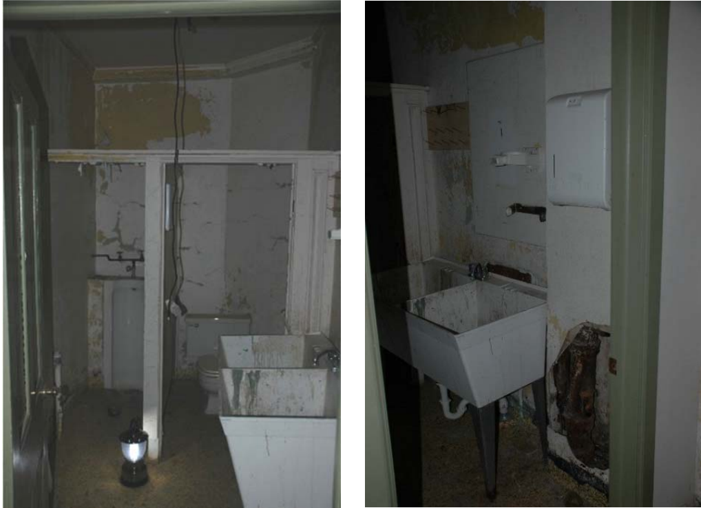
Figure 1.3-34: Views of Room 113 looking east (left) and looking southeast (right).
