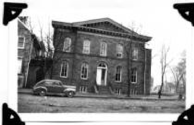
Figure 1.2-67: State Insurance Survey dated 1941 identifies the Sheriff's House as the New Castle Club. The description indicates that renovations and redecorating had taken place within the last few years. 77
