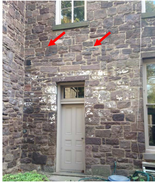
Figure 1.2-32: (Upper Right) A line of mastic above the west door and traces of whitewash around the door opening define the dimensions of a former structure. Whether this was a connector to the prison as shown on the 1885 plan or simply a later porch has not been determined. (Upper Left) The mastic line continues around onto the courtyard wall. (Lower Left) A closed window opening is visible in the north side of the courtyard wall.
