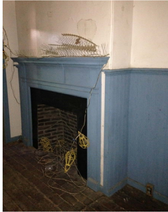
Figure 1.2-61: (Left) Wainscot was installed over the original wall plaster in the southwest kitchen c. 1915-1920. (Right) This fireplace was likely built c. 1920 after the original fireplace on the south wall was removed.
