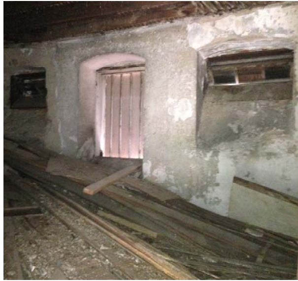
Figure 1.3-15: (Left) Original window openings survive in the north wall of the prison; (Right) Seen from the interior, these openings contain metal grilles. The smaller openings are also equipped with sashes.
