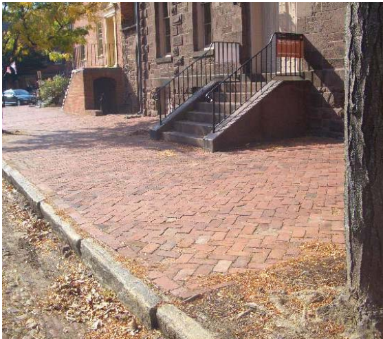
Figure 1.5-3: (Left) The brick-paved walking surface in front of the Sheriff's House is in good condition despite settlement of individual bricks. The surface is generally level with minor lipping. (Right) Tree roots have dislodged bricks in their immediate vicinity as well as some curb stones.
