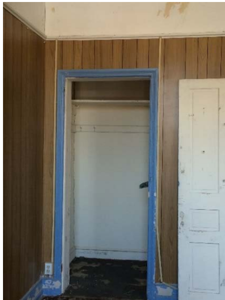
Figure 1.3-42: Views of Room 206 looking south (top left), looking east (top right) and looking west at existing closet (bottom left).
