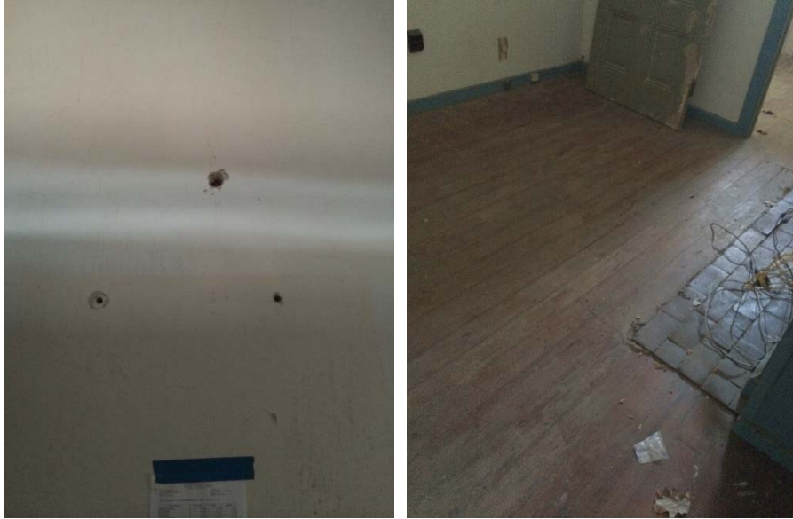
Figure 1.5-32: View of fastener damage at east wall (left) and flooring wear (right) in Room 109.
