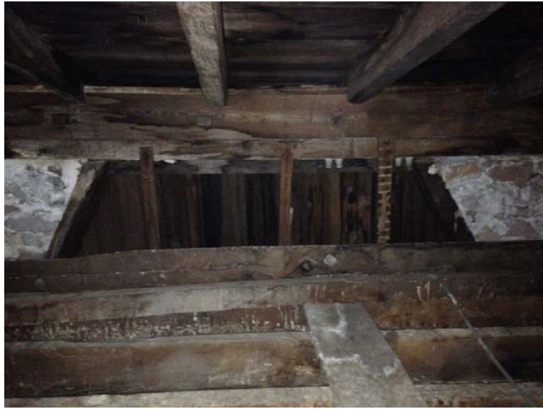
Figure 1.2-11: A sloped opening in the north wall of the attic corresponds to where the north end of the 1857 structure intersected the gable roof of the earlier sheriff's house which remained in place until the 1793 jail could be removed.
