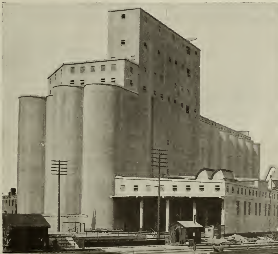
WASHBURN-CROSBY ELEVATOR AT MINNEAPOLIS
