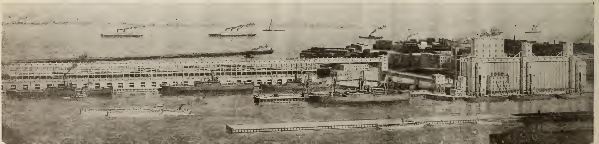
New York State Barge Canal Terminal Elevator Now Under Construction
