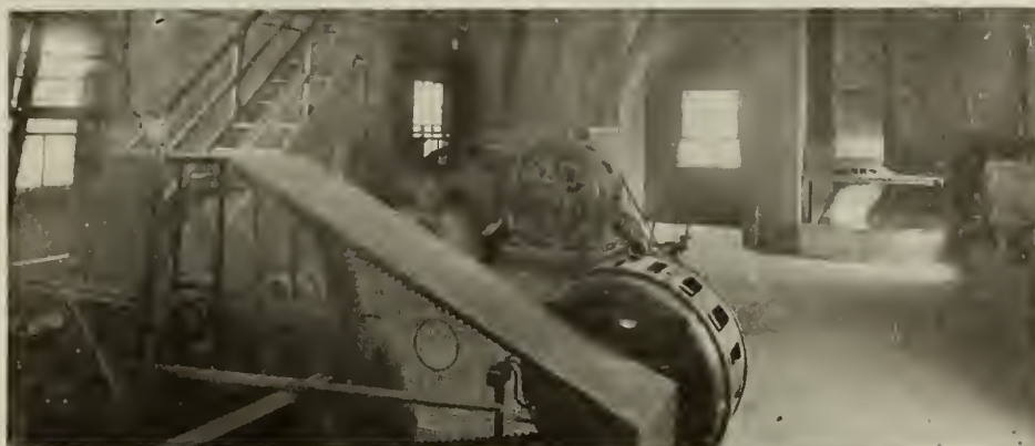
MORSE CHAIN DRIVE IN WASHBURN-CROSBY ELEVATOR
