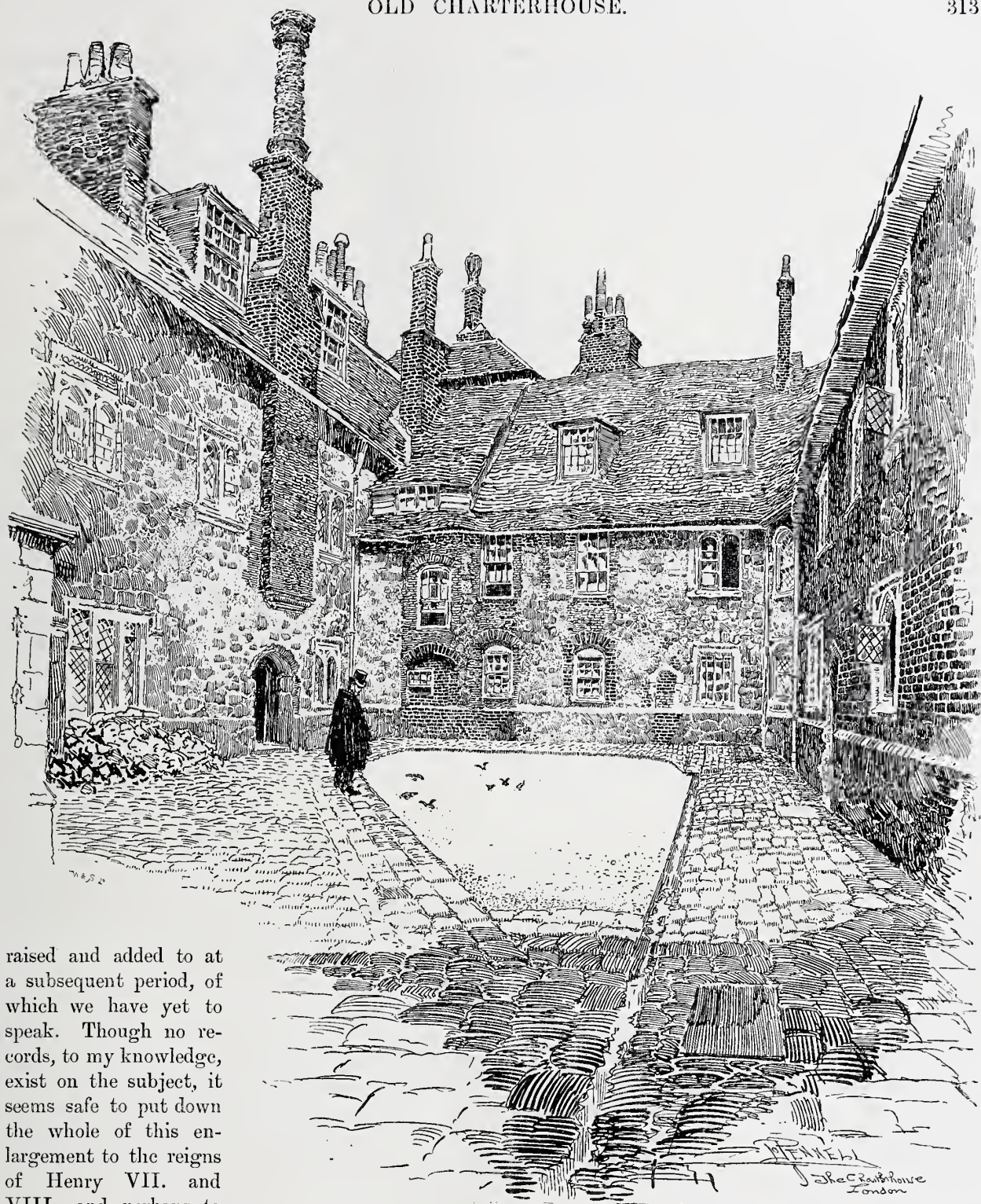
IV. — IN WASHHOUSE COURT.
