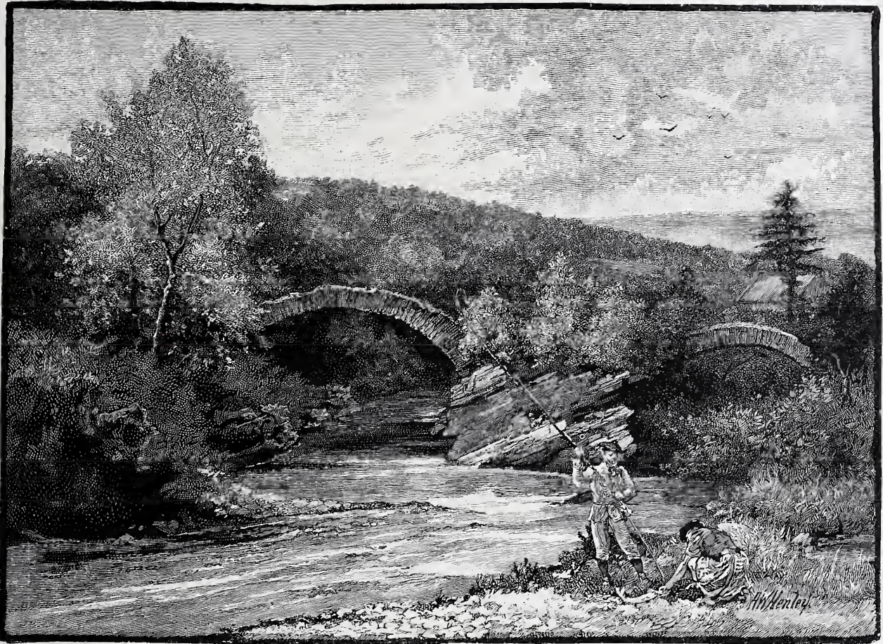
V.—GENERAL WADE'S BRIDGE.
