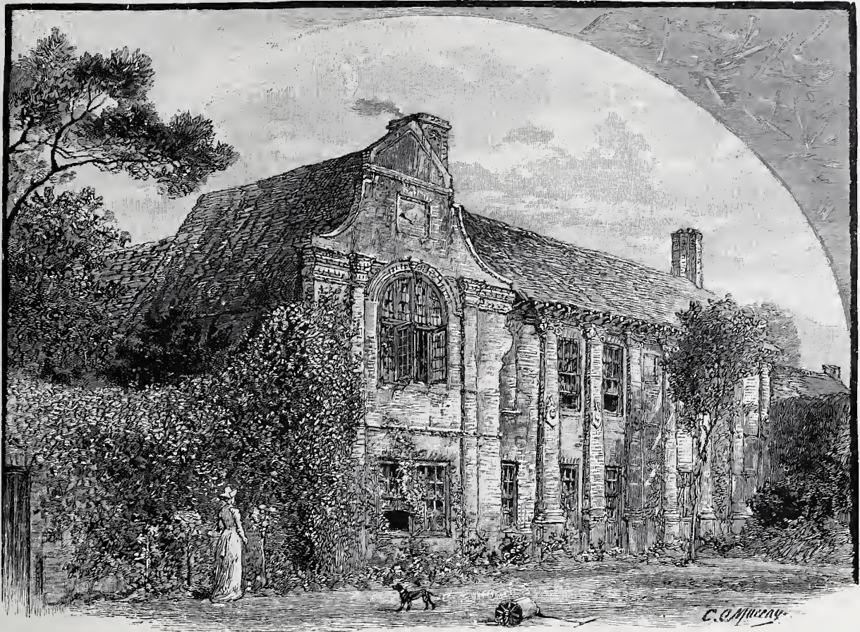
I.—SLYFIELD HOUSE: THE GARDEN FRONT.
