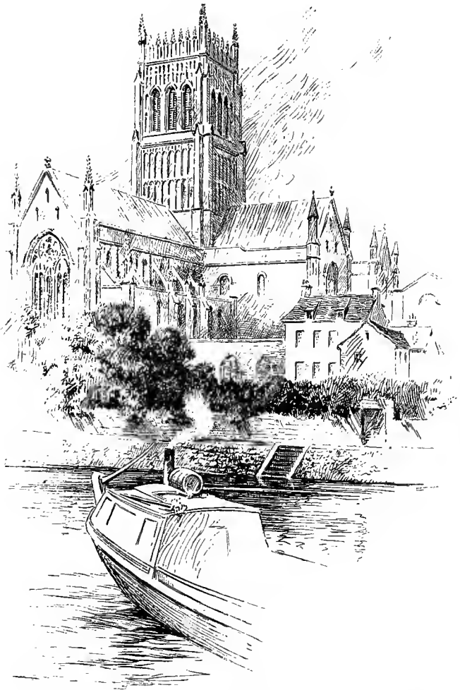
WORCESTER CATHEDRAL FROM THE SEVERN
