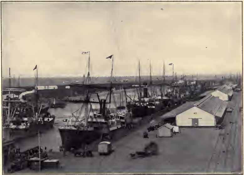
One of the basins in the Buenos Aires docks.
