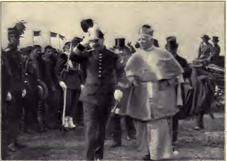
President Montes and the Archbishop just after turning the first shovelful of earth on the new railway.
