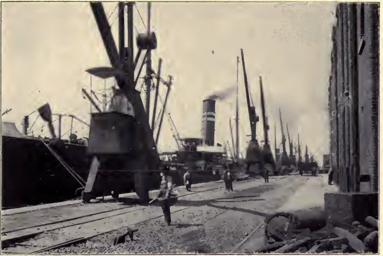
Cranes used in loading and unloading ships at the Buenos Aires docks.
