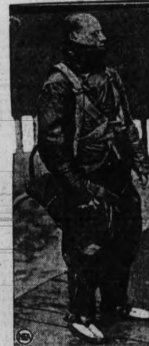
SAFETY FIRST! —Funny looking outfit this man is wearing. It's a new life preserver for army and navy aviators flying across water. The suit is lined with padded kapoc, a French material that is much lighter than water.
