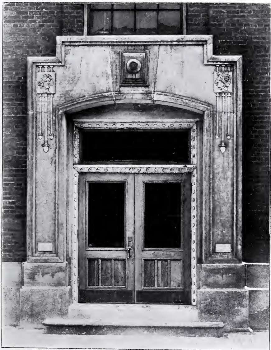
FIG. 5. THE INDIANA AVENUE ENTRANCE TO PASSENGER ELEVATORS AND PUBLIC STAIRS—BUILDING OF THE EASTMAN KODAK COMPANY.
