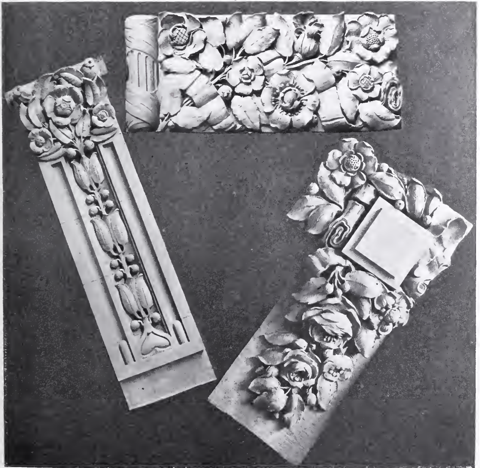
DETAILS OF WHITE SEMI-GLAZE TERRA COTTA.
