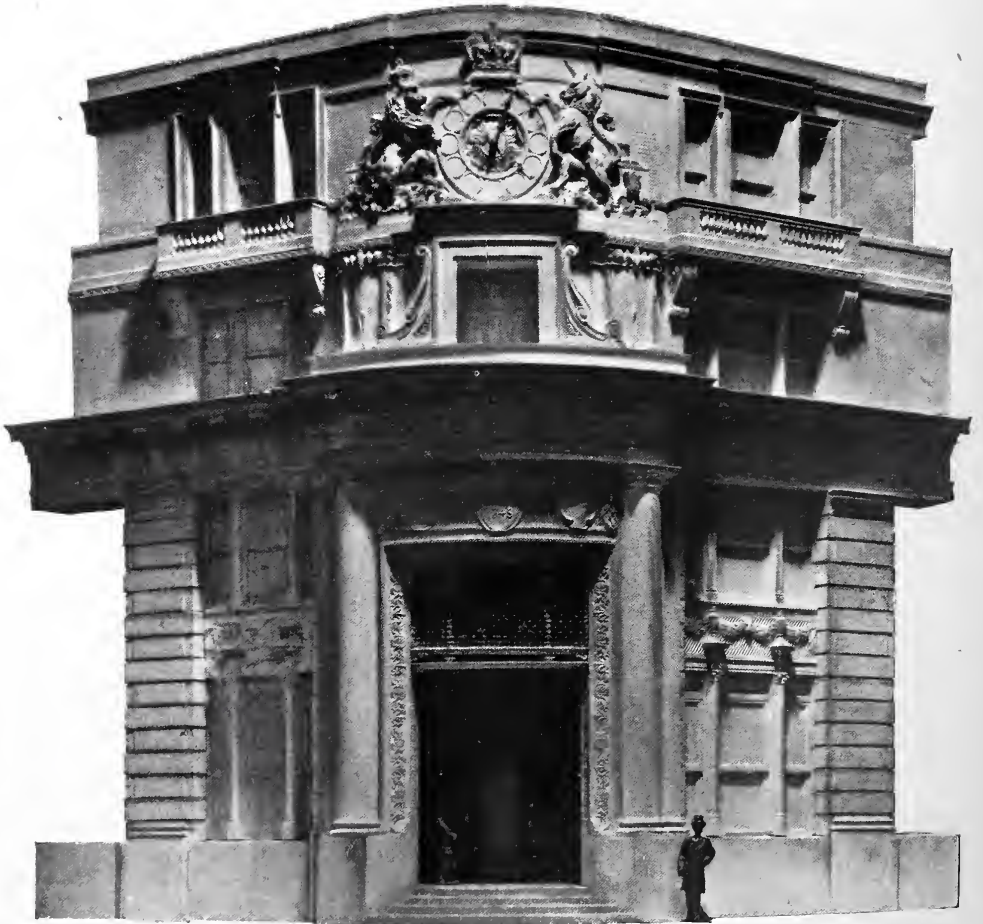
DETAIL OF THE ENTRANCE—ROYAL INSURANCE BUILDING.
