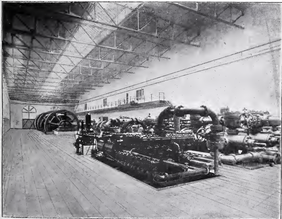
ENGINE AND PUMP ROOM—SEARS, ROEBUCK & CO. BUILDINGS.
