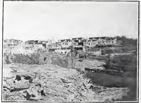
Fig. 5. Laguna Pueblo Houses Built of Stone, from which the Plaster has Fallen.
