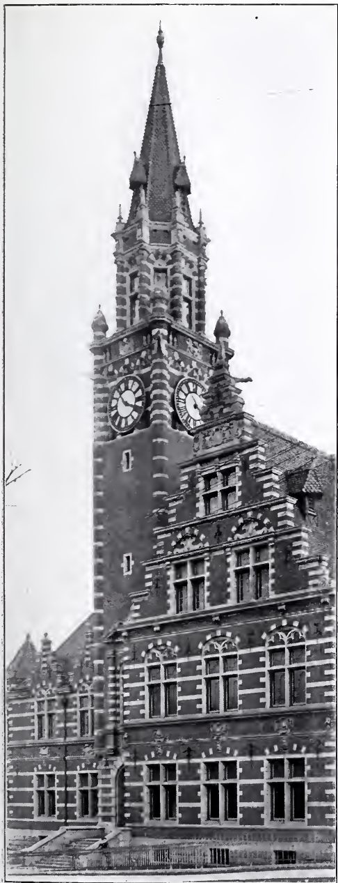
FIG. 3. THE TOWER OF THE POST OFFICE. Paterson, N. J.
