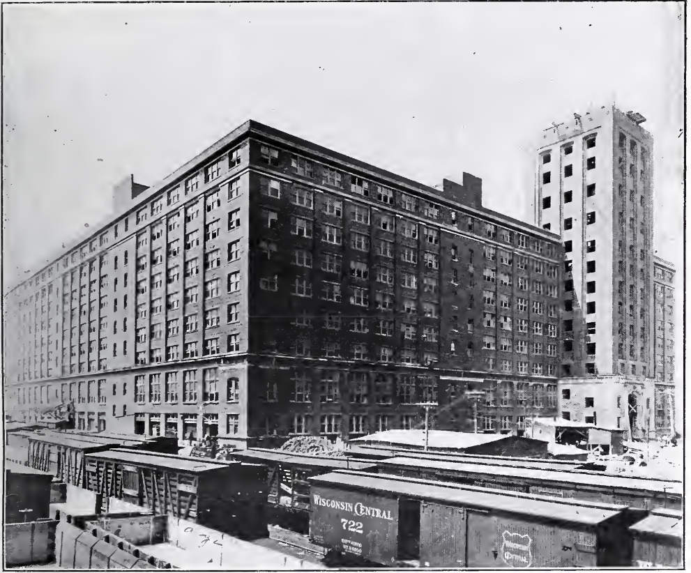
MERCHANDISE BUILDING, LOOKING NORTHWEST—SEARS, ROEBUCK & CO.
