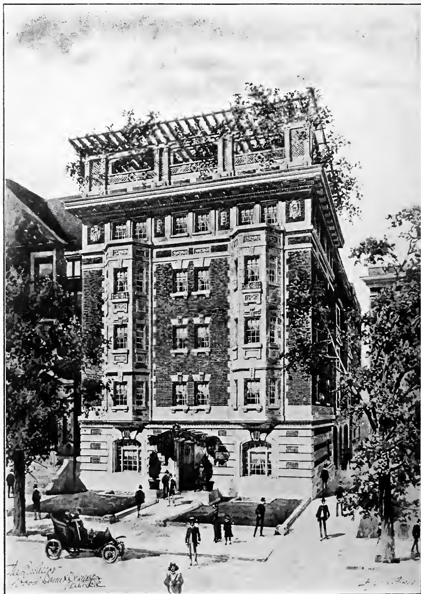
"THE BACHELOR" APARTMENT HOUSE.
