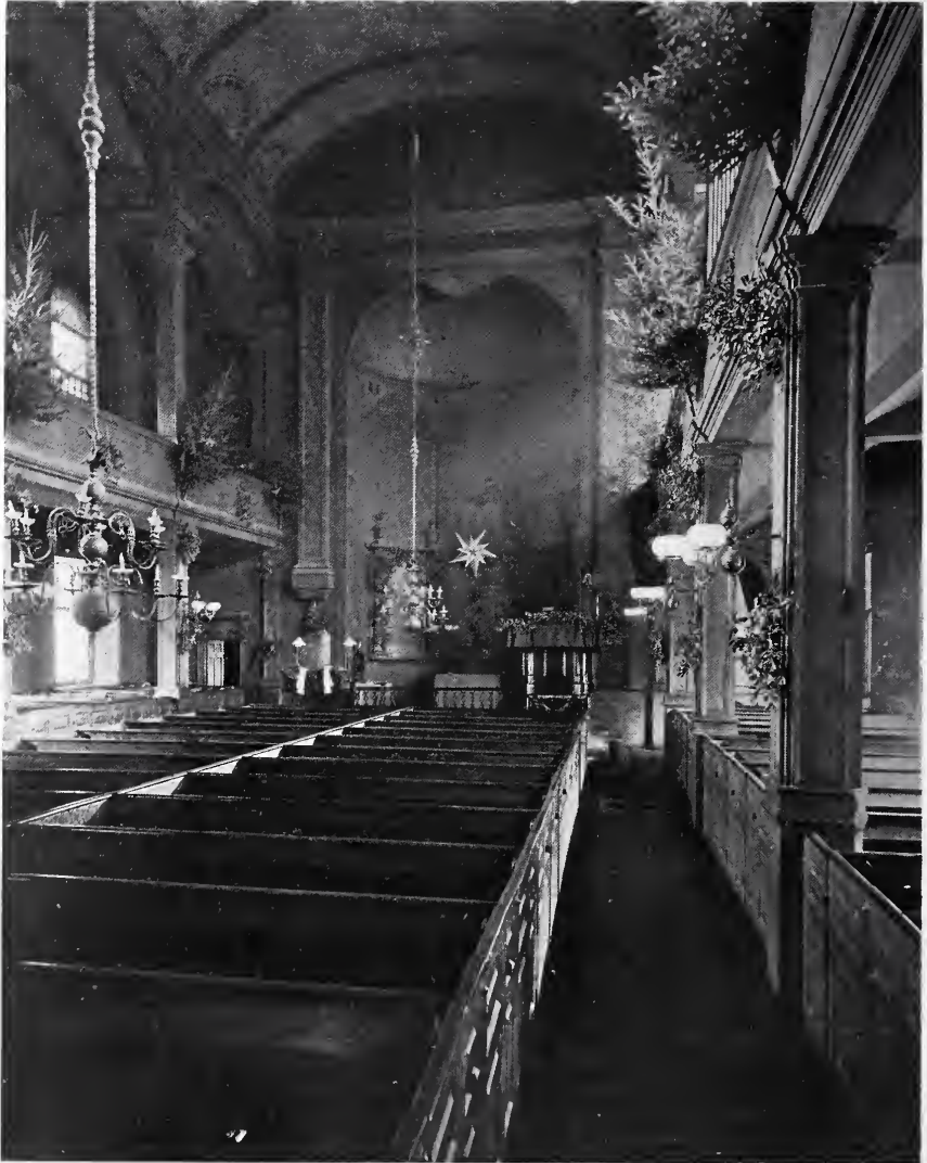
FIG. 2. GENERAL VIEW OF THE INTERIOR OF NORTH CHURCH.
