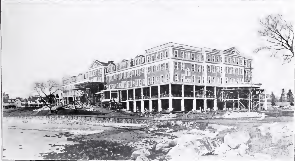
1. NORTHWEST WING AND MAIN BUILDING. 2. FROM THE SOUTHWEST.
