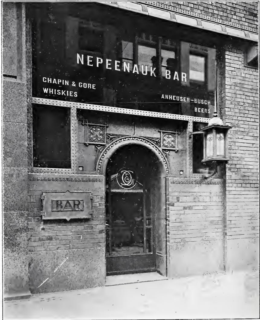
FIG. 4.—ENTRANCE TO BAR IN THE CHAPIN & GORE BUILDING.
