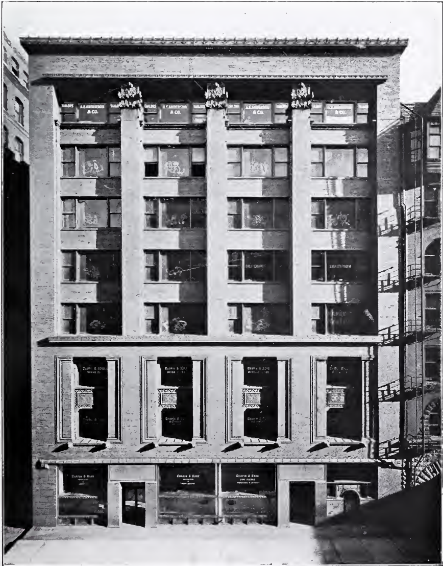
FIG. 3.—THE CHAPIN & GORE BUILDING.
