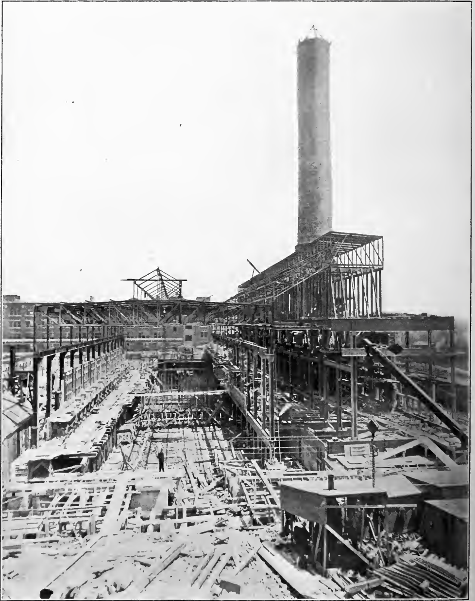
CONSTRUCTION OF THE POWER HOUSE—SEARS, ROEBUCK & CO.
