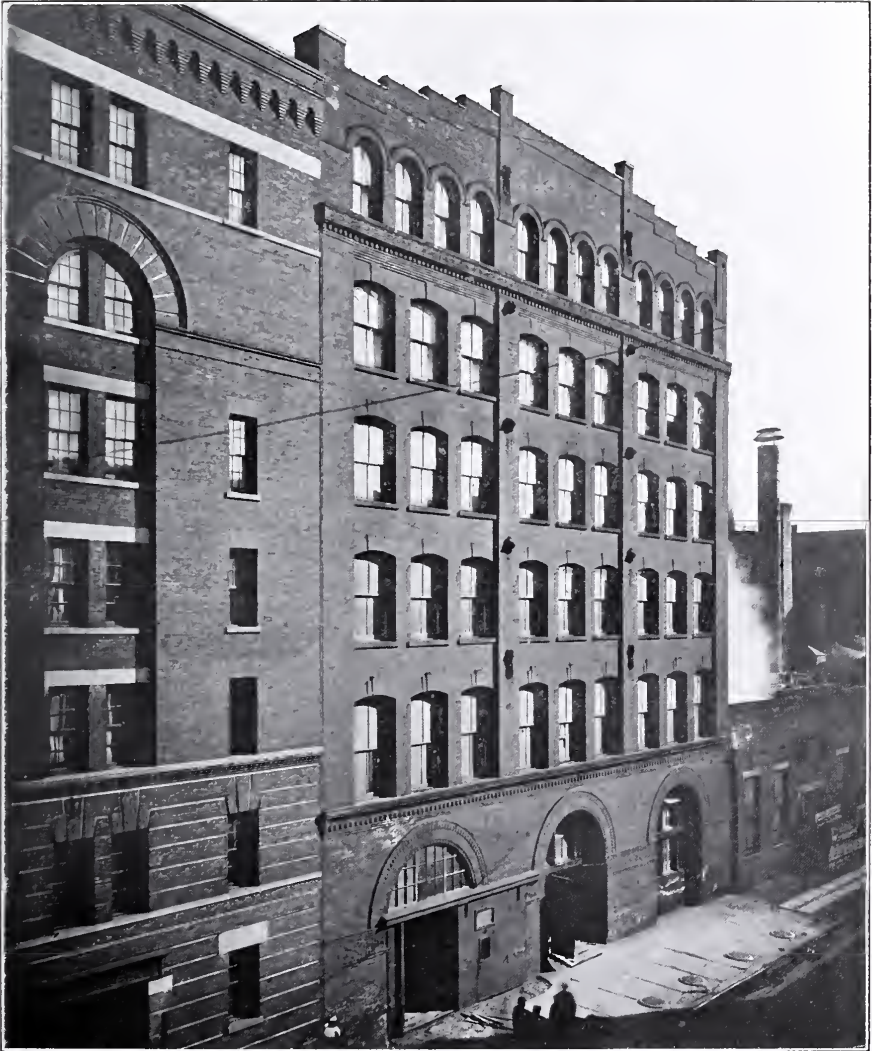
FIG. 2.—WAREHOUSE OF I. T. WILLIAMS & SONS.
