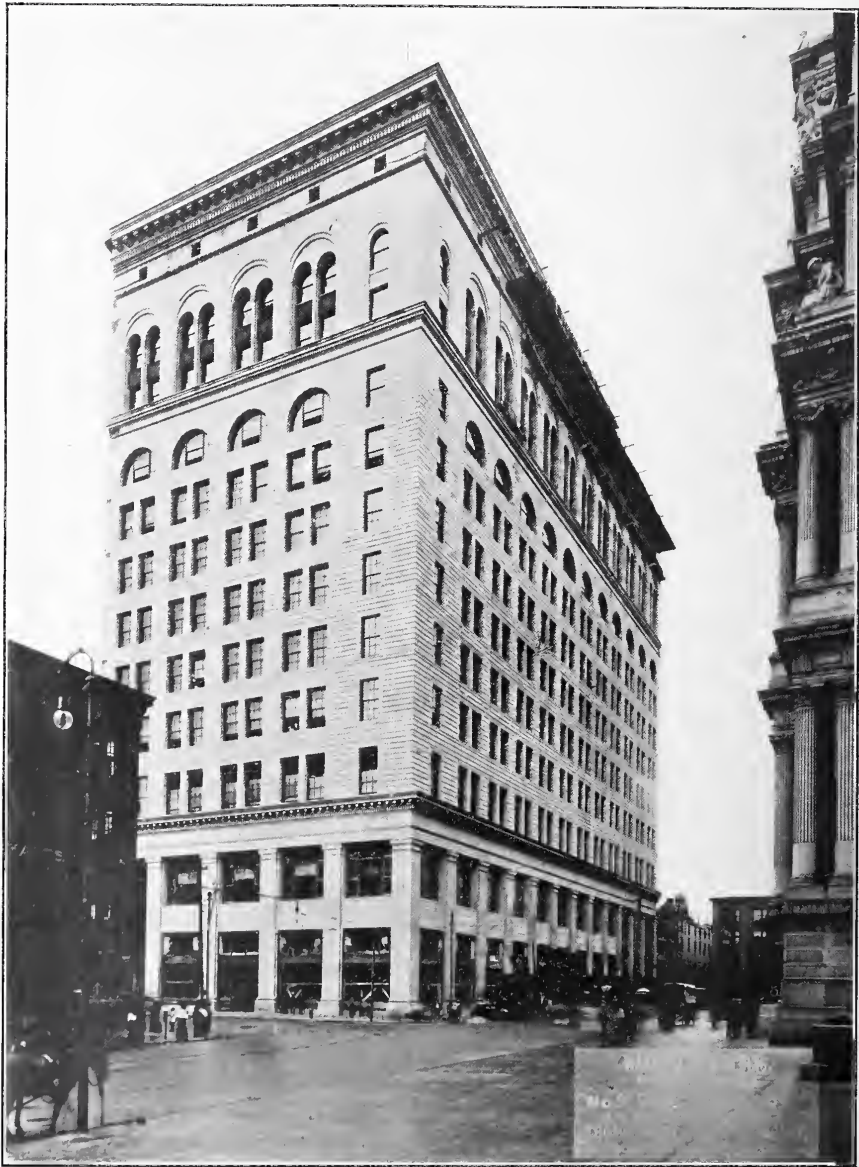
THE NEW WANAMAKER BUILDING.
