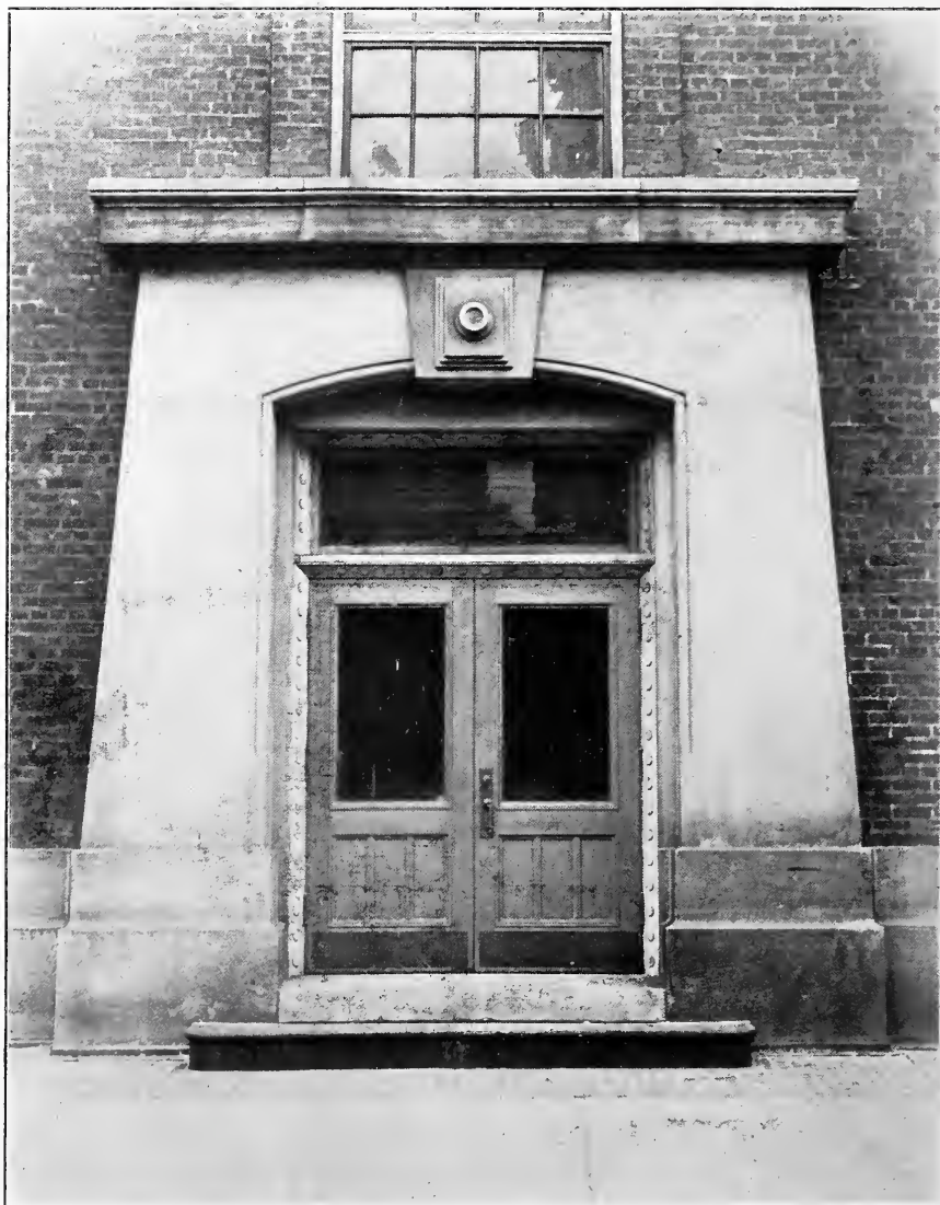
FIG. 6. THE SERVICE ENTRANCE ON 18TH STREET—BUILDING OF THE EASTMAN KODAK COMPANY.
