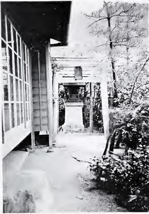
Fig. 3. The side of this house shows the way in which the posts rest upon exposed stones, which are slightly hollowed to receive them.
