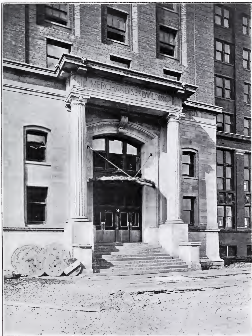
THE MAIN ENTRANCE TO THE MERCHANDISE BUILDING.
