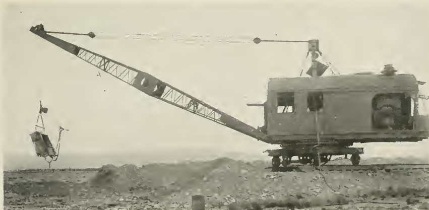
A PAIR OF FLYCATCHERS BUILT THEIR NEST AND REARED THEIR YOUNG AT THE PLACE MARKED X IN THE ARM OF THIS DREDGE WHILE IT WAS IN OPERATION
