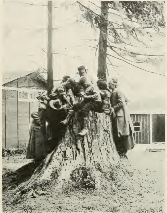
DR. C. F. HODGE HELPING SOME OF THE BOYS OF THE MULTNOMAH CLUB BUILD A CEMENT BIRD-BATH IN A STUMP.
